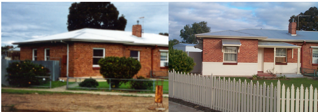
Figure 6.9: Renovation of SAHT Dwelling, The Parks
