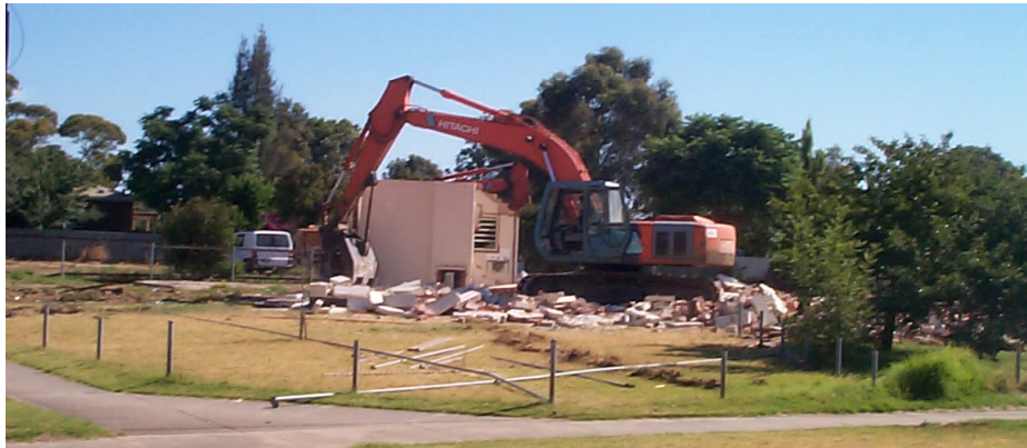
Figure 6.8: Demolition of SAHT Dwelling, The Parks
