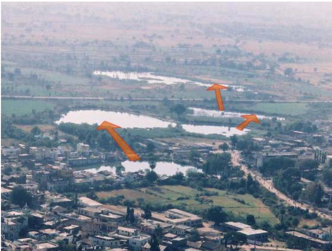
Figure 5.5: Aerial photograph of connected tanks (Author 2008)
