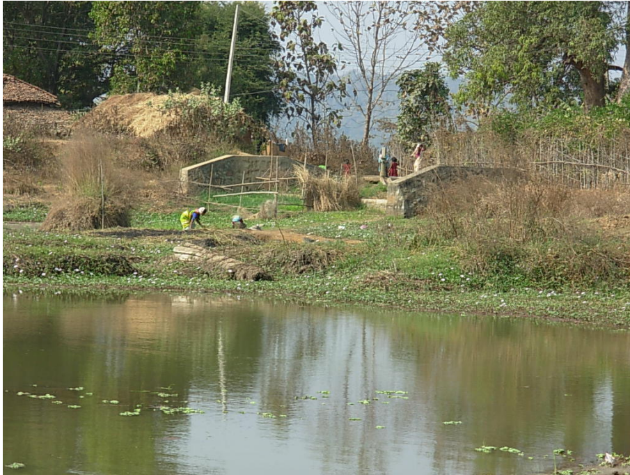
Figure 6.16: Photograph of tank and waste weir (Author 2008)
