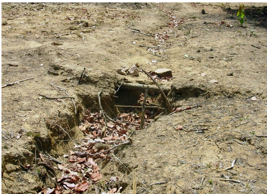
Figure 6.8: Photograph of check-dam across a seasonal forest stream (Author 2009)
