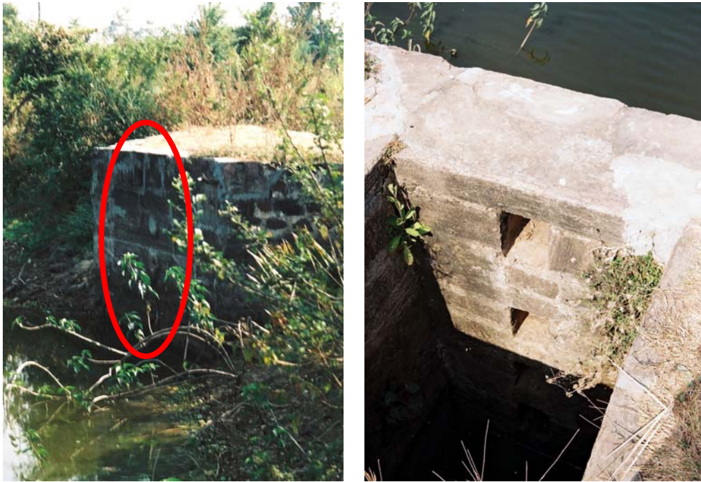
Figure 5.8: Photographs of an overflow system using stone structure (Author 2008)
