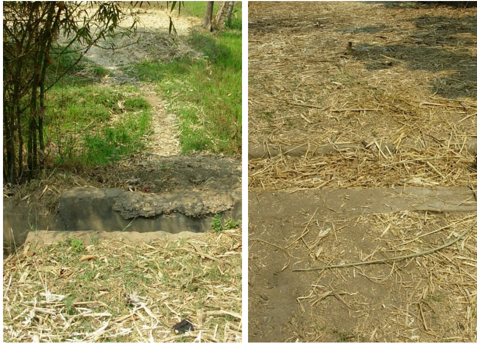
Figure 6.20: Photographs of encroached and neglected pats (Author 2009)
