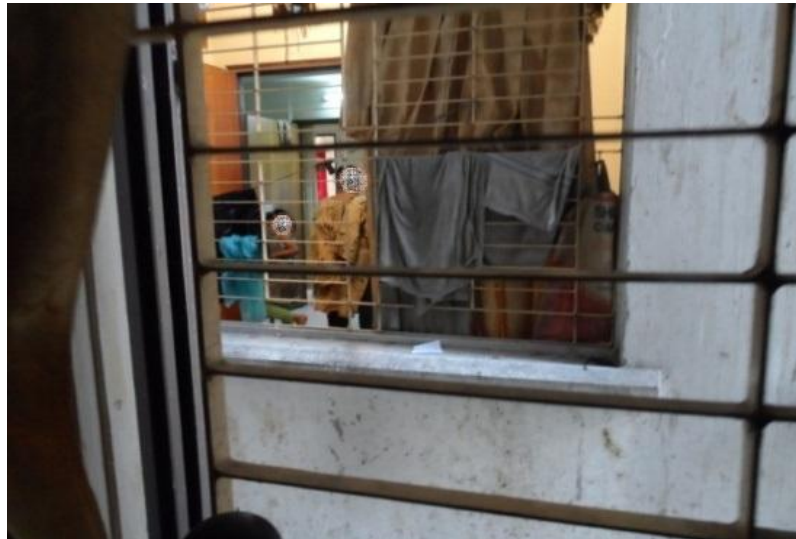
Figure 6-23: Low setback distance between buildings causing lack of visual privacy
