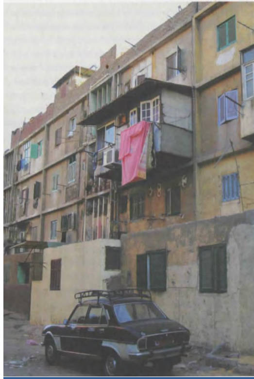
Figure 20. Public Housing in Imbaba.
