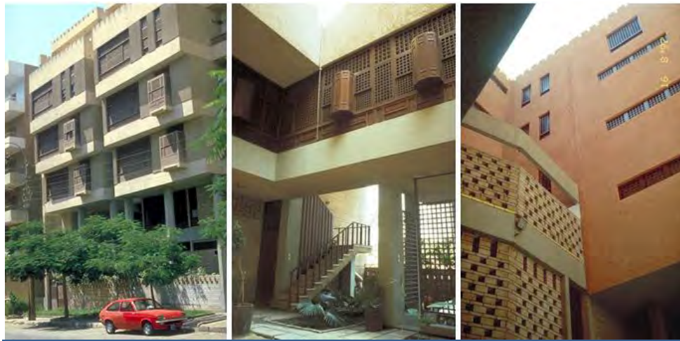
Figure 81. The CPAS Façade and Central Courtyard.
