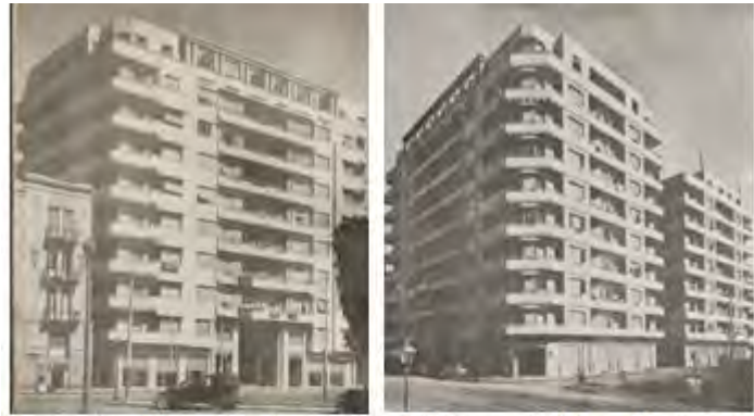
Two facades of Bahari, the intersection of Muhammad Mahmud St., built in 1934 (1939, no. 10). Note the horizontal ornamented stripes around balconies as well as the floral decorative top.
