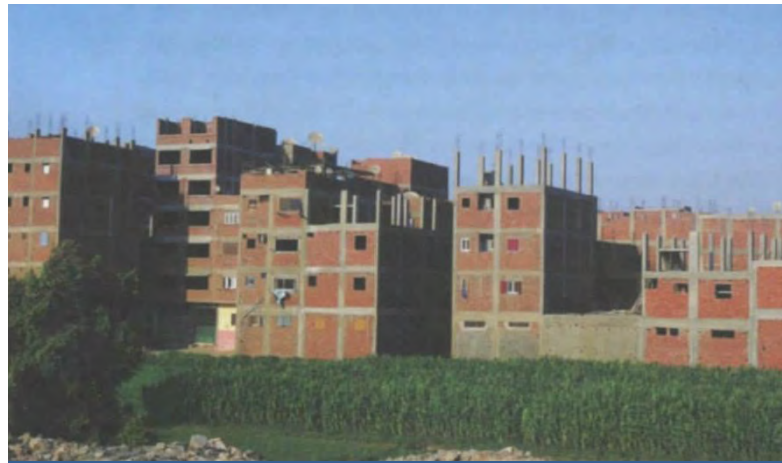
Figure 25. Unauthorized Settlement on Agricultural Land.
