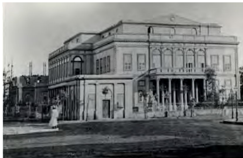
The main façade with a tripartite volume composition, and Ionic columns. A statue was made in the centre of the square of Ibrahim Pasha, Isma‘ail’s father, made by Charles Cordier (1872).
