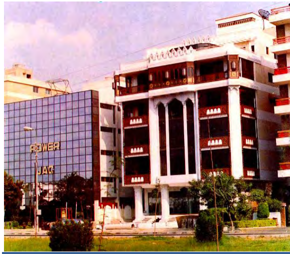
Figure 96. Contrasting Two Different Trends in Adjacent Buildings.
