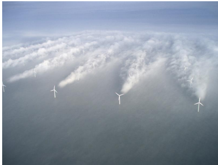
Figure 2.8 - The cumulative wake at the Horns Rev 1 in Denmark, illustrating the severity of conditions at a typical wind farm (Owned by Vattenfall. Photo rights owned by Christian Steiness).
