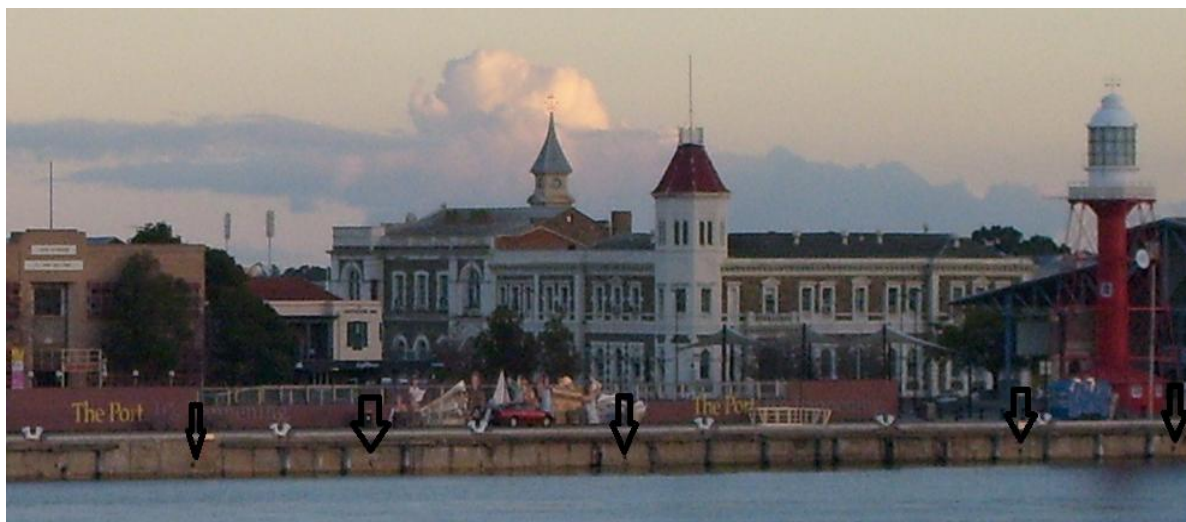
Figure 4.17 McLaren Wharf: outlets of storm water drainage network
