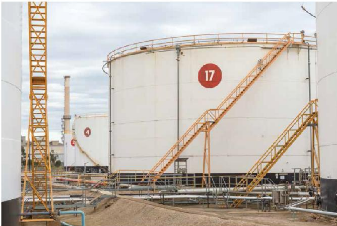
Figure 6.7 Large-sized petrol tanks at Birkenhead Terminal
