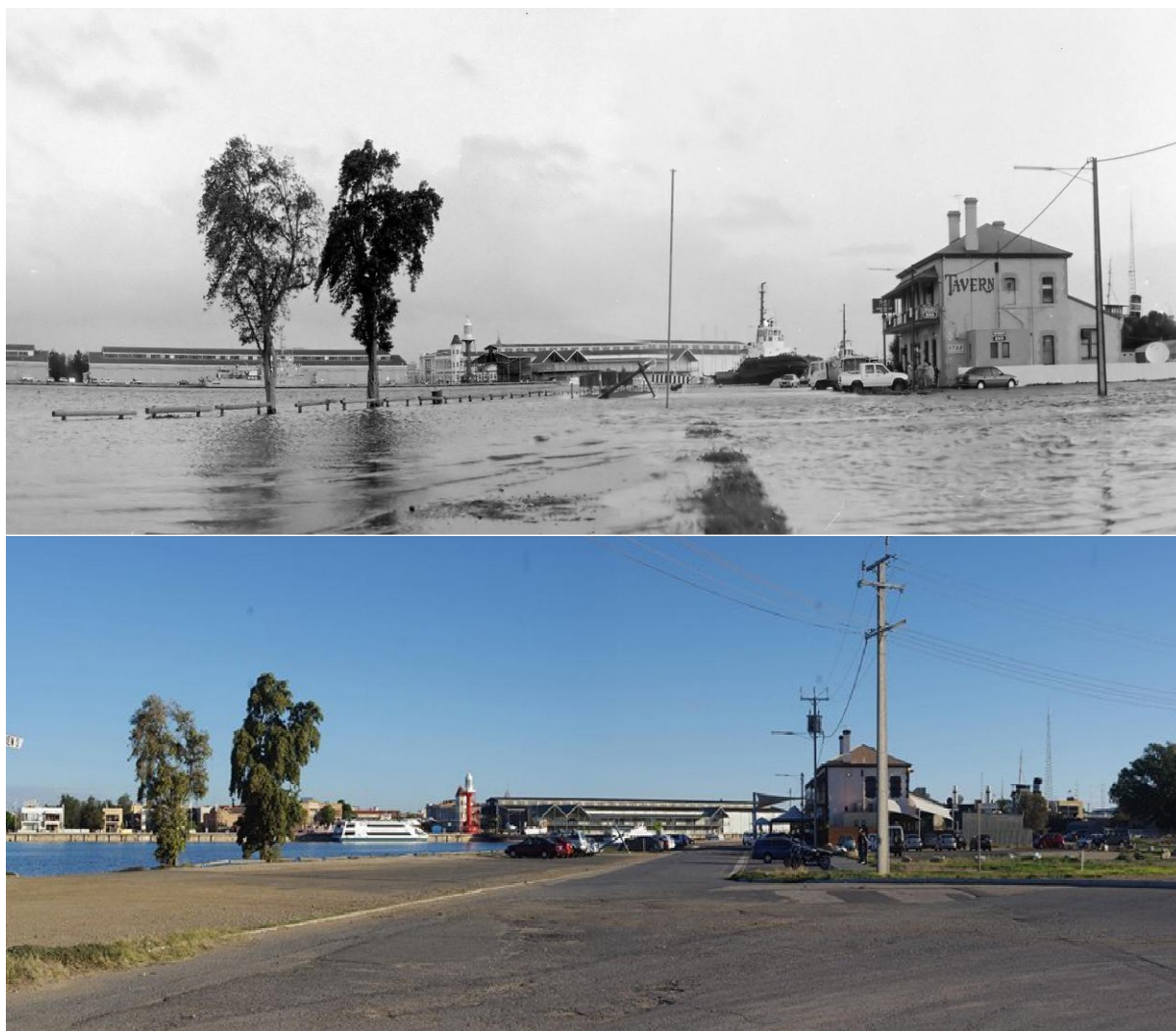
Figure 4.8 Flooding at Birkenhead Tavern in July 1995 (top photo)
