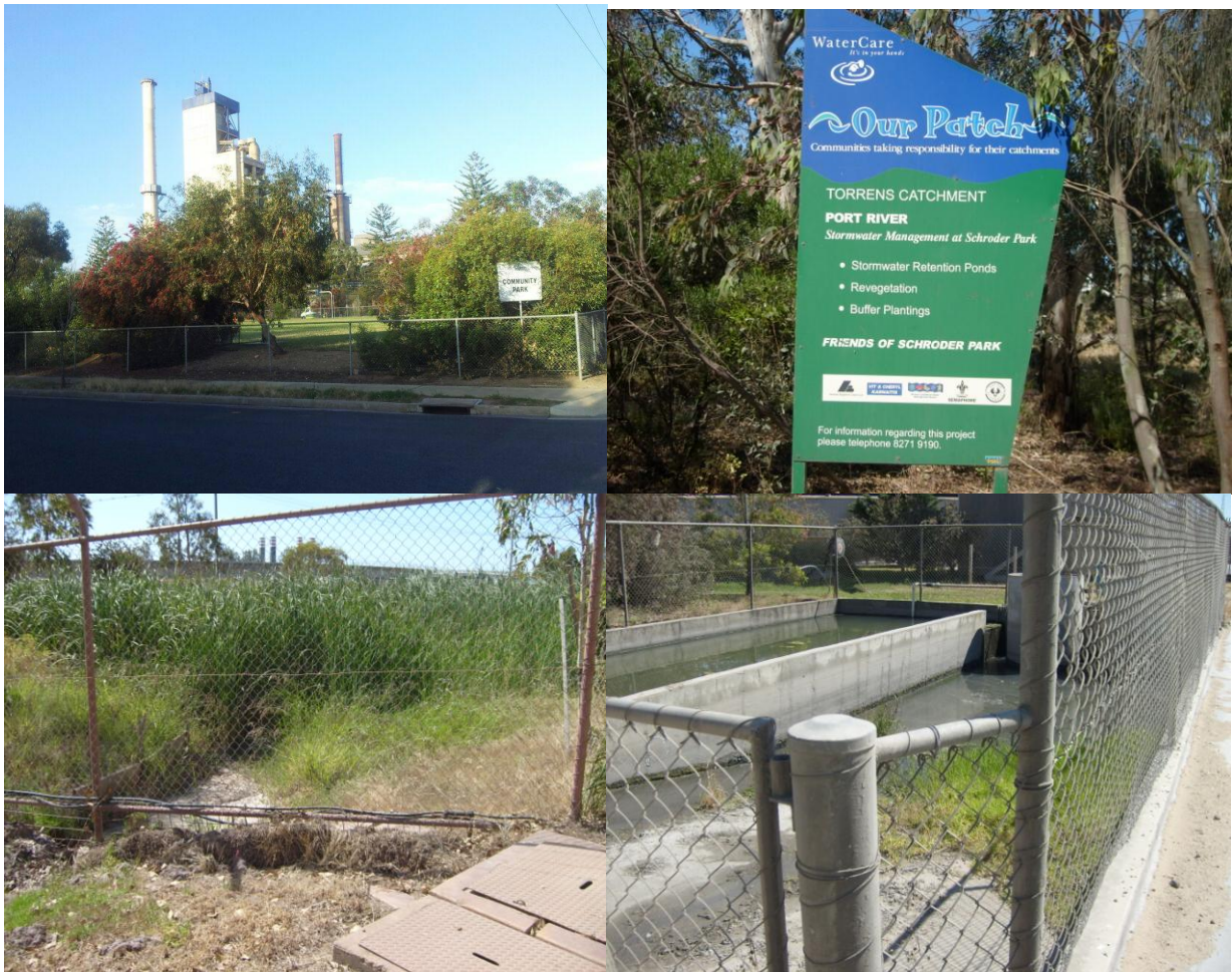
Figure 6.10 ABC’s storm-water capturing systems
