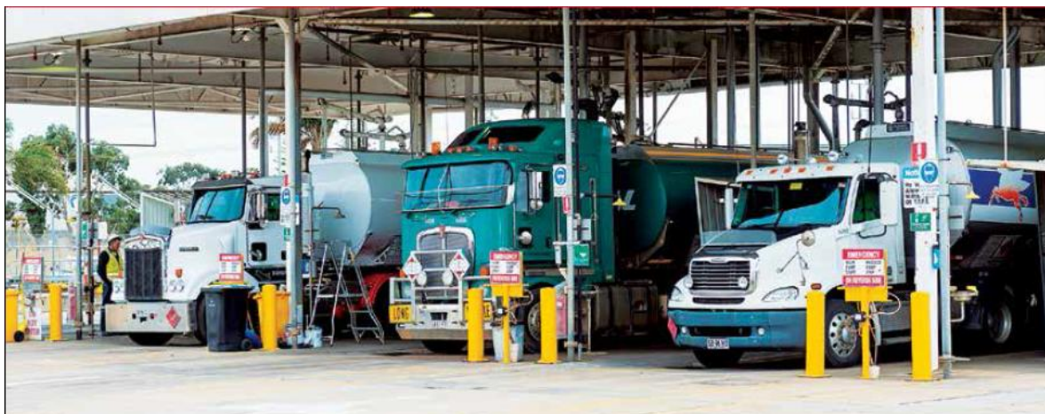
Figure 6.6 Loading tank trucks at the Birkenhead Terminal
