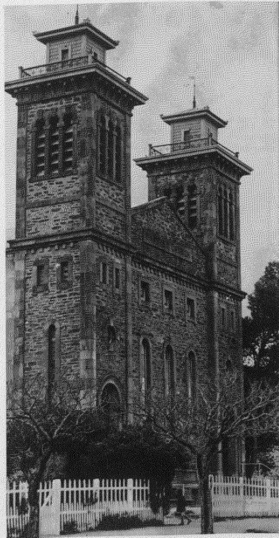
The Baptist Church. Now an Adult Education Centre, this is the first and only building erected by the Baptists.
