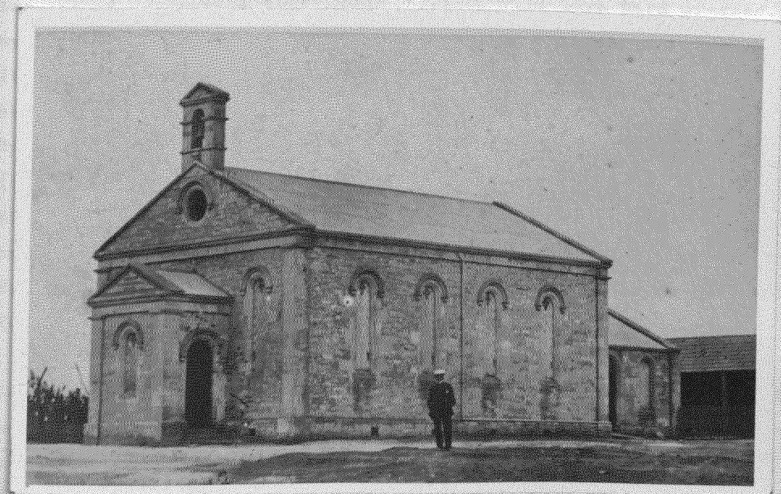
Congregational Chapel. It is very close to the mines and the old manager's house - the first minister was also mine manager.
