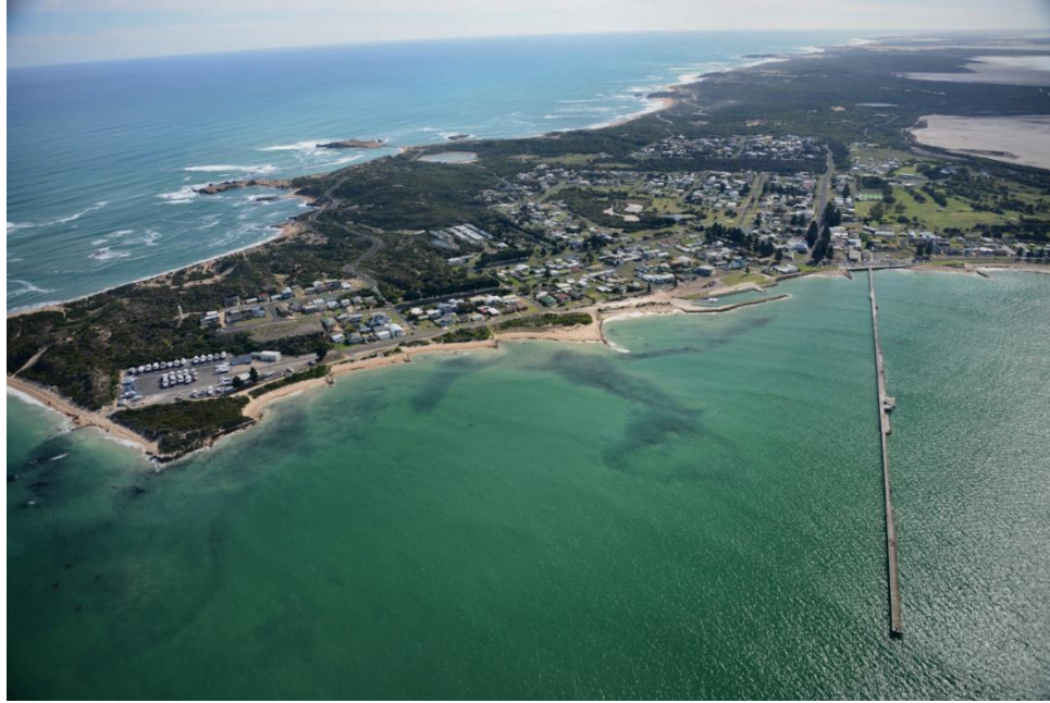
Figure 5.17 Aerial photograph of District Council of Wattle Range coastline
