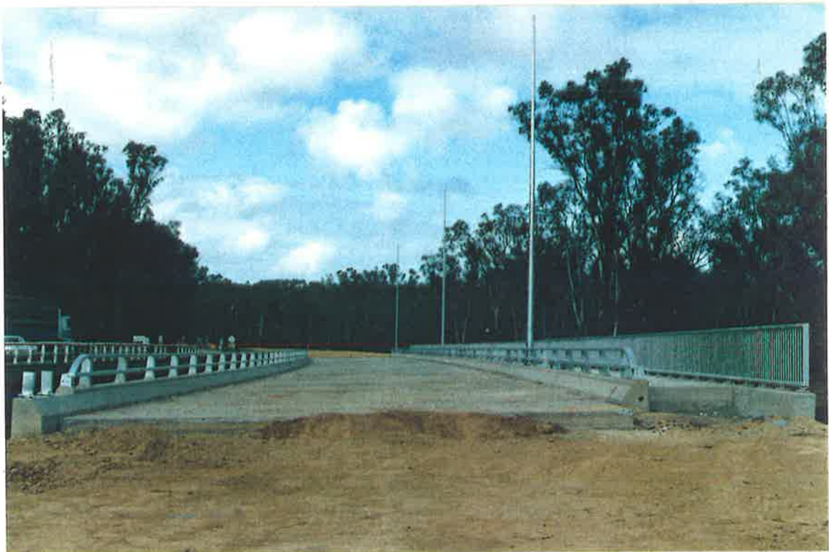
Plate 1.2: Composite bridge prior to placement of asphalt
