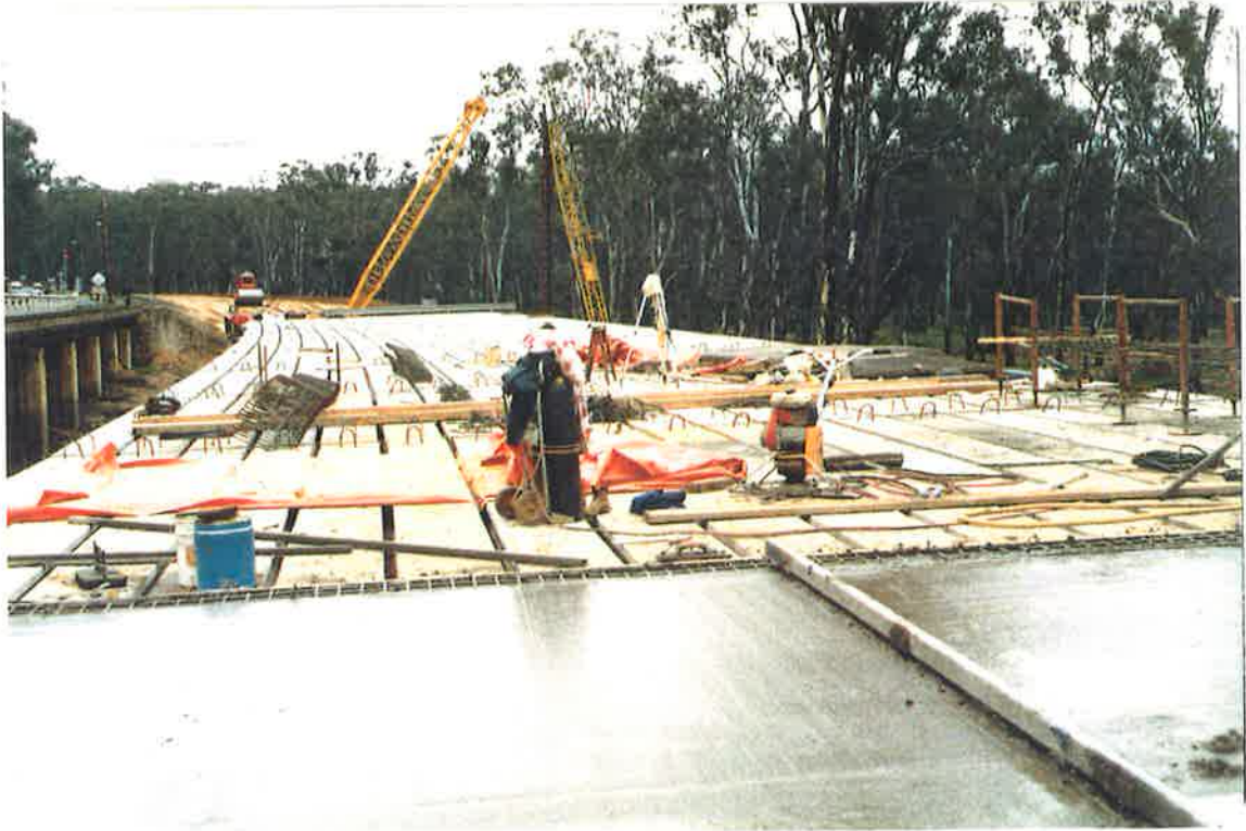
Plate 1.1: Composite bridge during the pour of the topping slab
