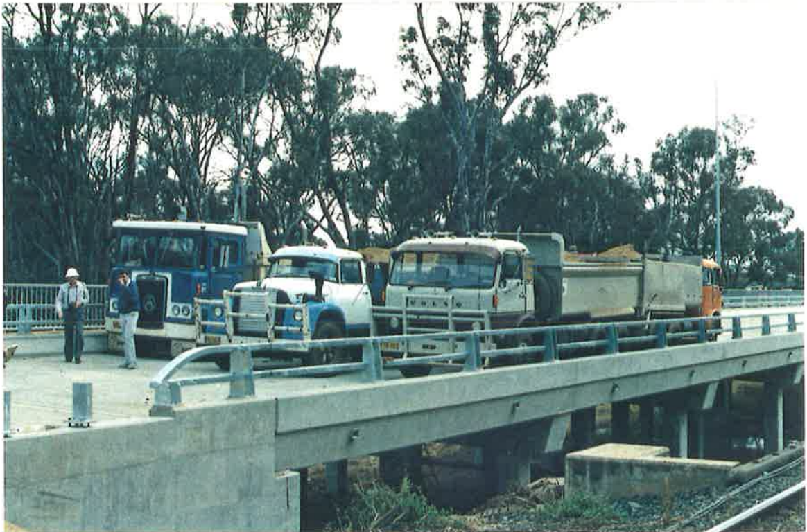
Plate 6.1: During test loading of bridge - Pattern #1
