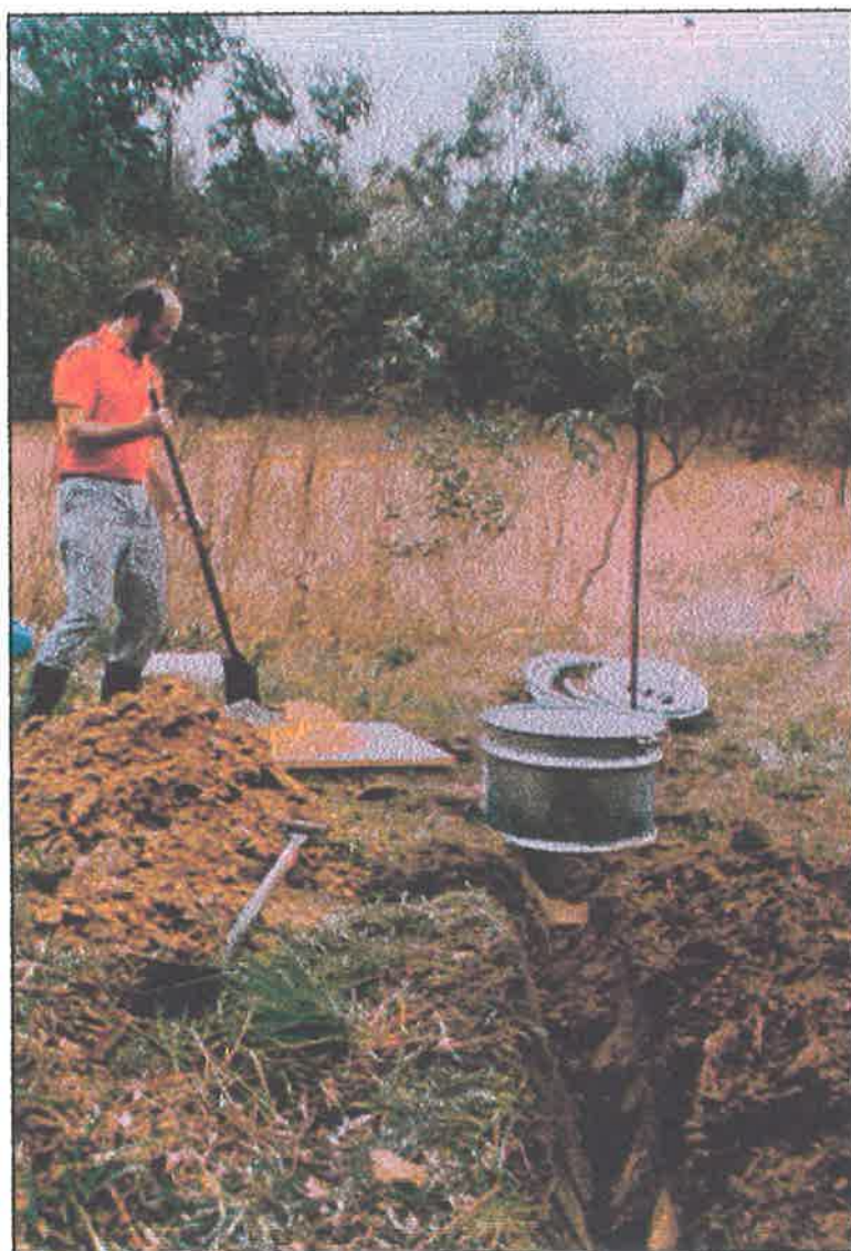
Figure 4-2 : Installation of the protective housing for the Inlet sampler
