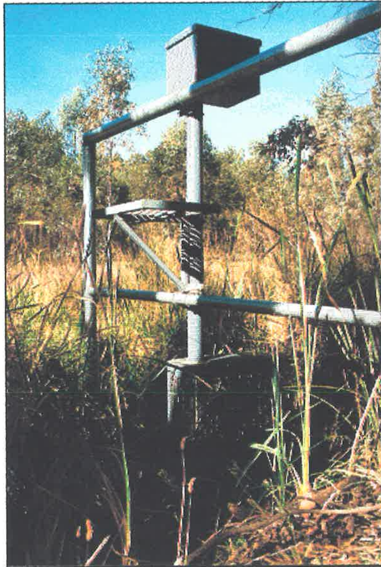
Figure 4-9 : Inlet station, instrument protective housing and intake structure
