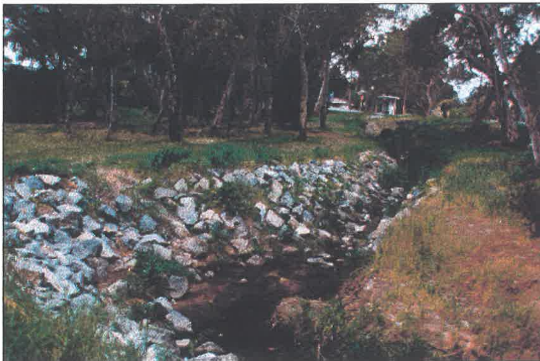
Figure 3-5 : Rip-rap lined channel at stormwater outlet, 400m upstream from wetland
