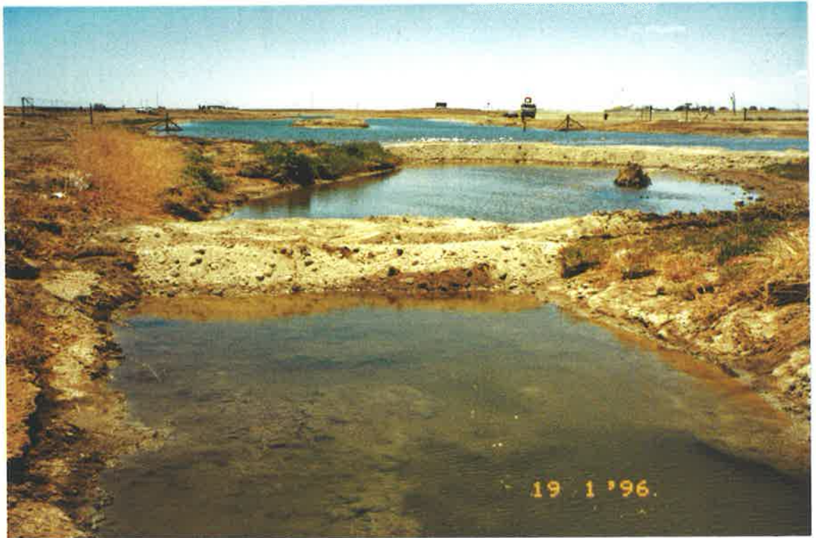
Photograph 4.4 Barker Inlet Wetlands during construction phase
