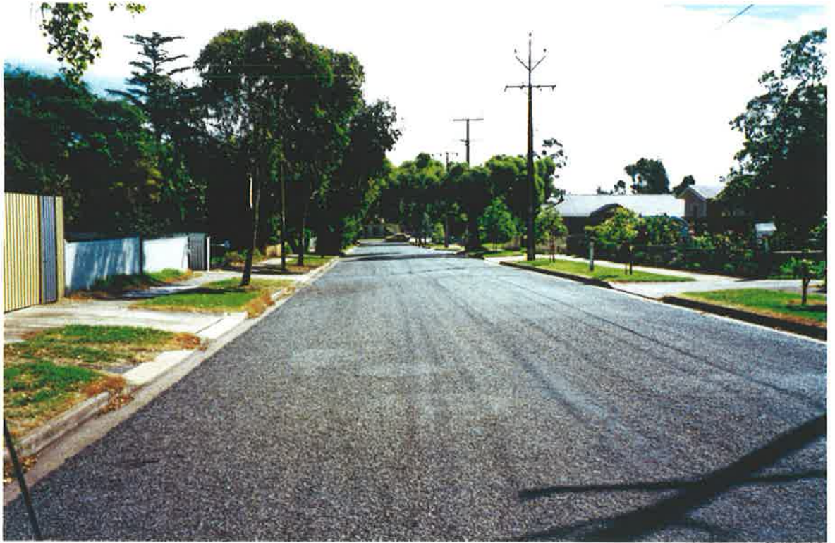
Photograph 4.3 McKay Street, Broadview – typical residential street in the North Arm East catchment.
