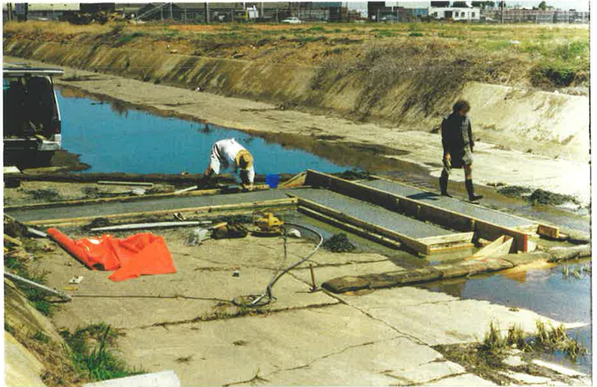
Photograph 4.14 The North Arm East monitoring station during construction
