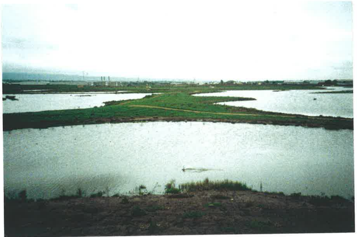
Photograph 4.5 Barker Inlet Wetland Southern Pond system shortly after completion. Pond 4 to left and Pond 3 to right, adjoining tailwater pond in foreground (photograph late 1996)
