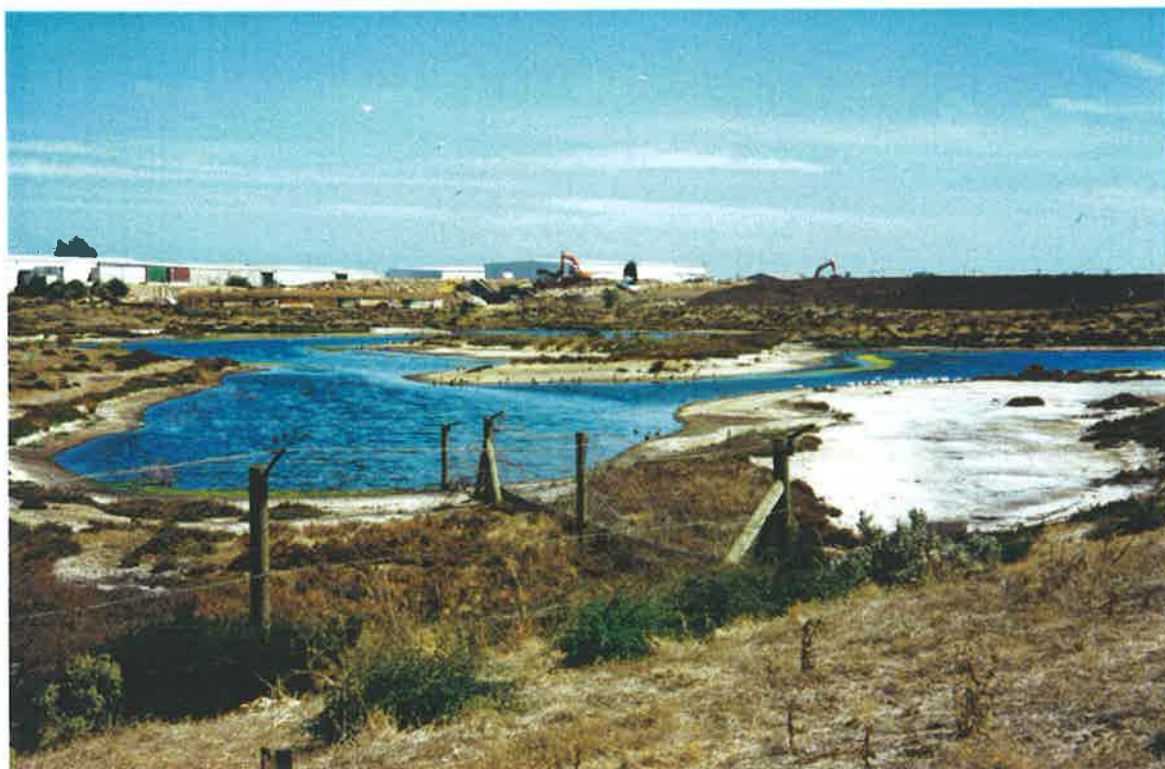
Photograph 4.9 Barker Inlet Wetland Pond 2. Little to no vegetation has established due to the visibly high salinity of the pond.
