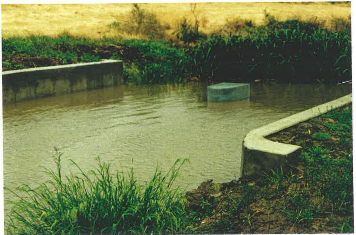
Photograph 5.12 The Henschke Street Drain during an event. There is no sign of the drowned out weir.
