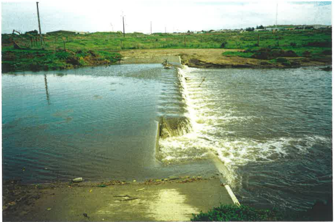
Photograph 6.1 Trashracks downstream of the North Arm East station full of litter during an event. Note that they are acting roughly as a broad crested weir.
