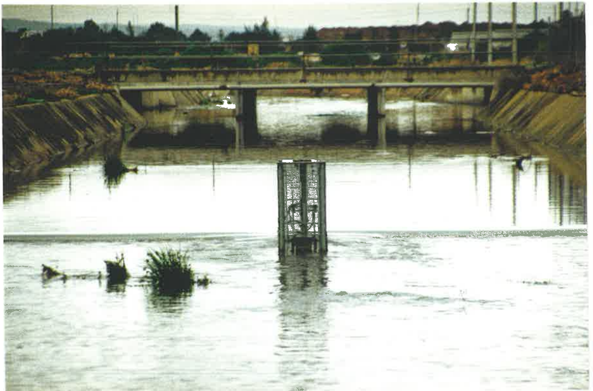
Photograph 4.15 The completed North Arm East monitoring station
