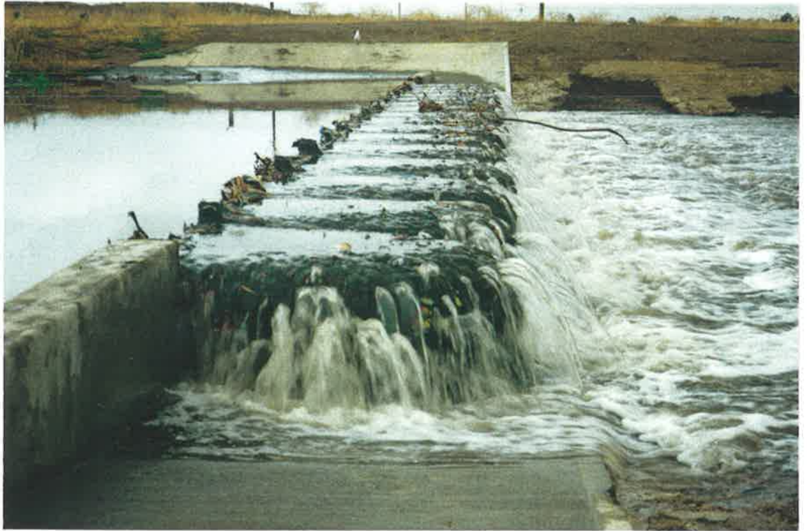
Photograph 5.6 Trashracks downstream of the North Arm East monitoring station full of litter during an event
