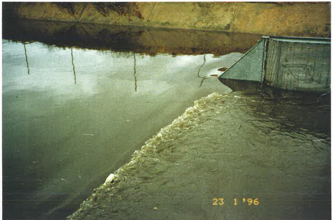
Photograph 5.7 North Arm East weir during an event prior to the installation of the trashracks. Note the head drop over the weir.
