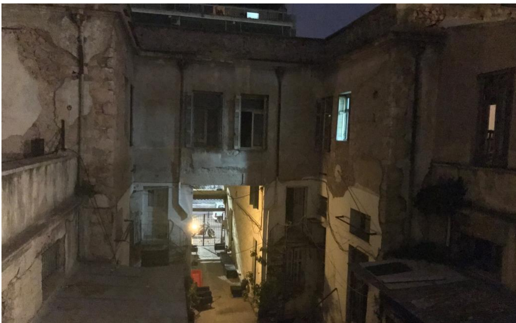
Figure 7.1 Derelict 1930s building used by Communitism, Metaxourgeio, Athens
