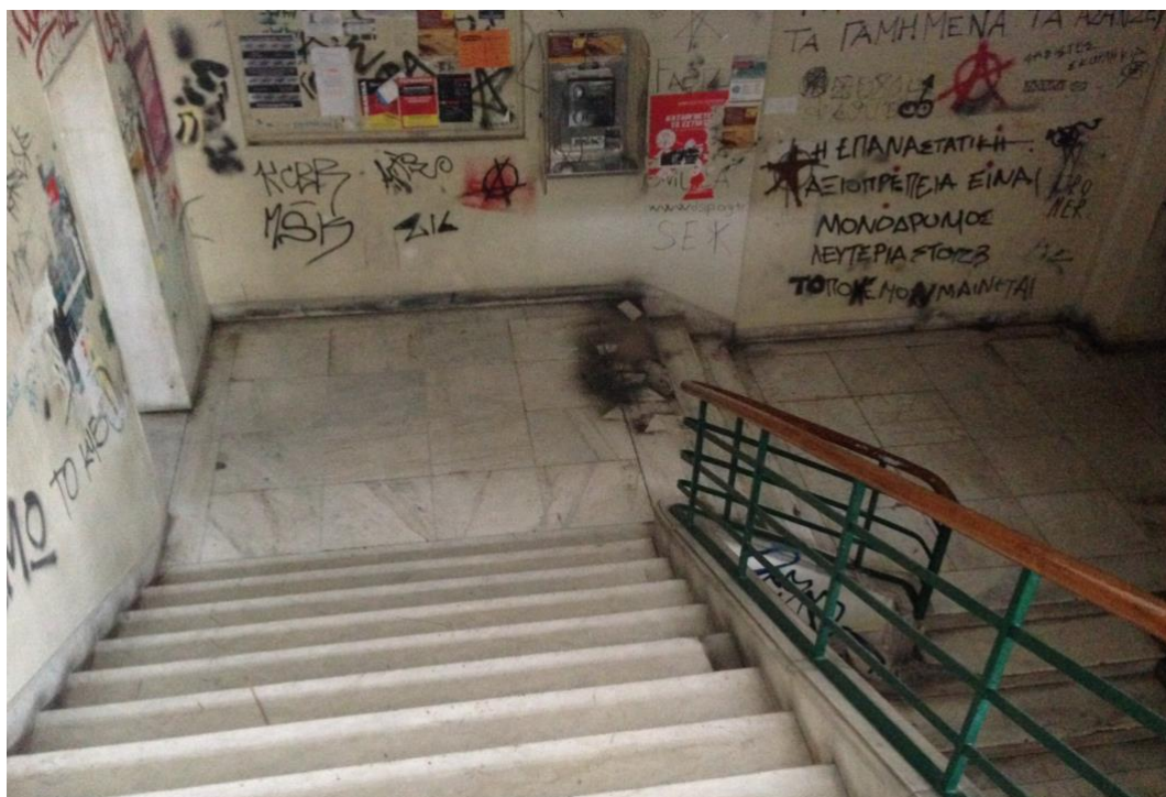
Figure 5.15 Athens Polytechnic stairwell
