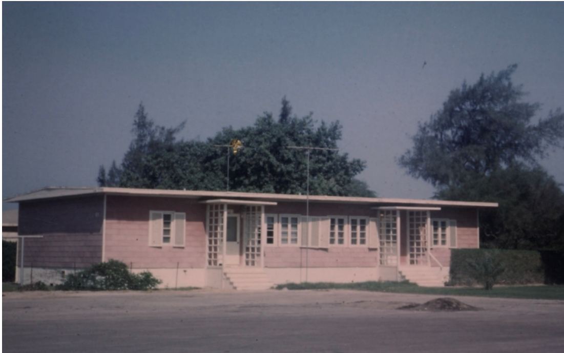
Figure 2.5 Swedish duplex after some modifications. The original external walls were covered in shingles. Photographer unknown. Courtesy of King Abdulaziz Foundation for Research and Archives (Darah).
