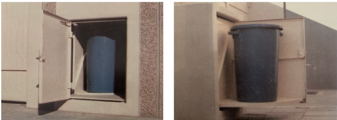
Figure 5.18 Waste bin box in the prefabricated villa boundary wall. Source: REDF Buraidah.
