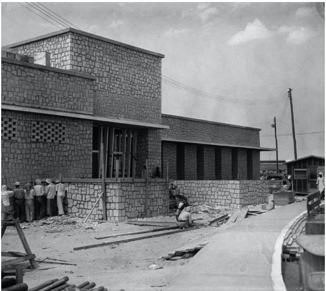
Figure 1.6 Italian workers completing stone facades of the Dhahran Dining Hall in 1948. Photograph unknown. Courtesy of Saudi Aramco.
