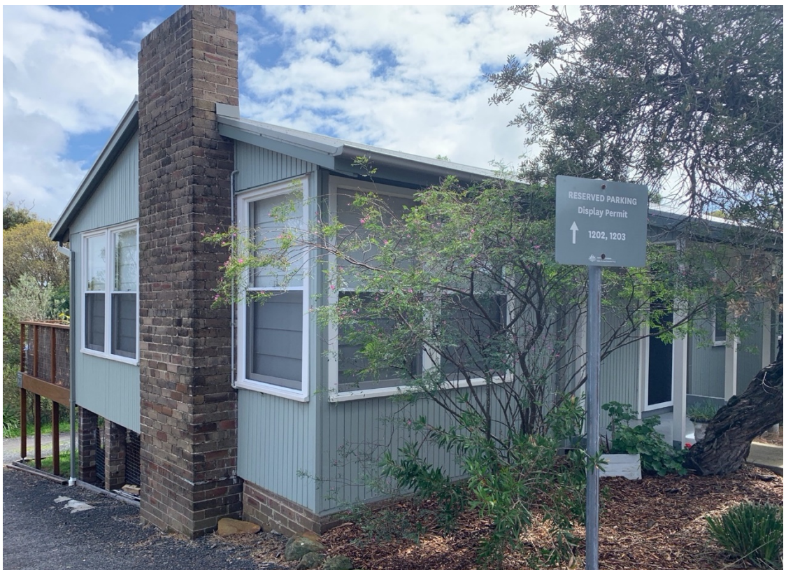
Figure 3.1 Above: One of the ASA Georges Heights houses in 2003 prior to restoration. Photograph: Roberson & Hindmarsh Pty. Ltd. Courtesy of Sydney Harbour Federation Trust. Below: One of the ASA Georges Heights houses photographed in 2019 following restoration. Photograph by authors.
