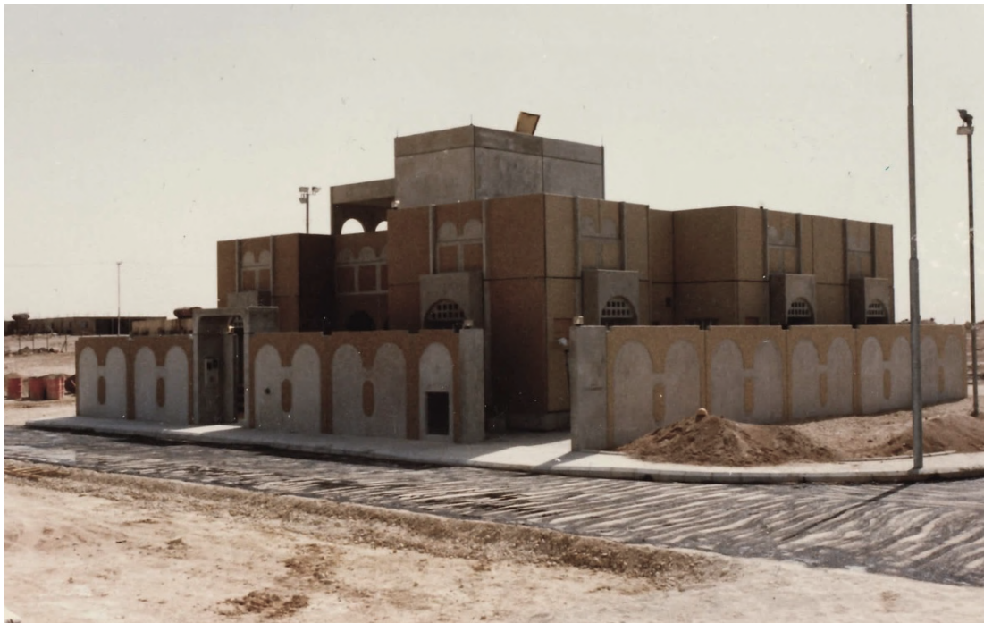
Figure 5.16 One of Buraidah’s prototype villas just after finishing assembly work. Source: REDF Buraidah.
