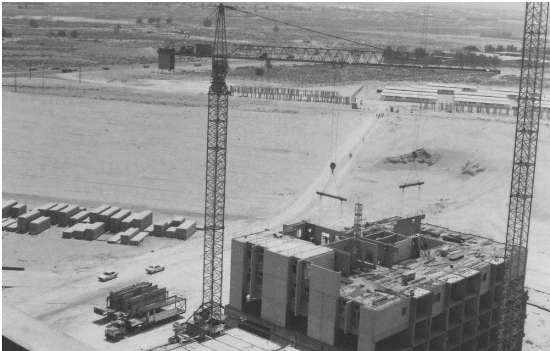
Figure 5.8 One of the towers under construction. Panels height and slabs are jointed at the floor level. Source: mapio.net
