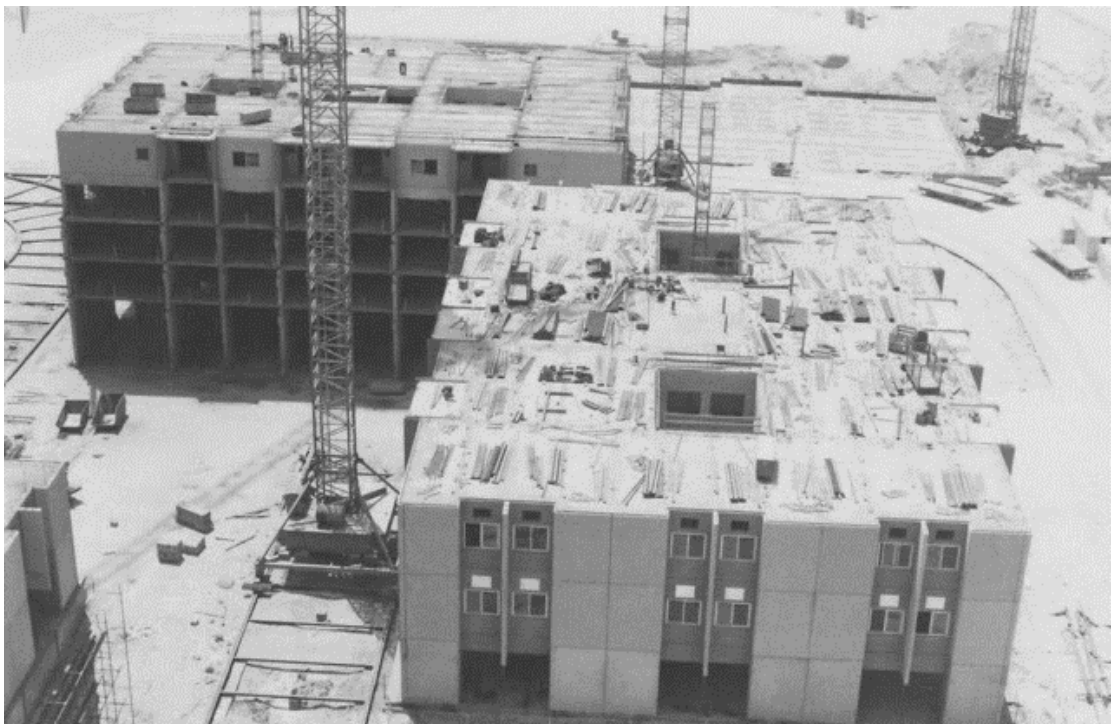
Figure 5.9 Temporary crane track. Above: the track was constructed from early on. Below: crane sitting on the track during construction. Source: mapio.net
