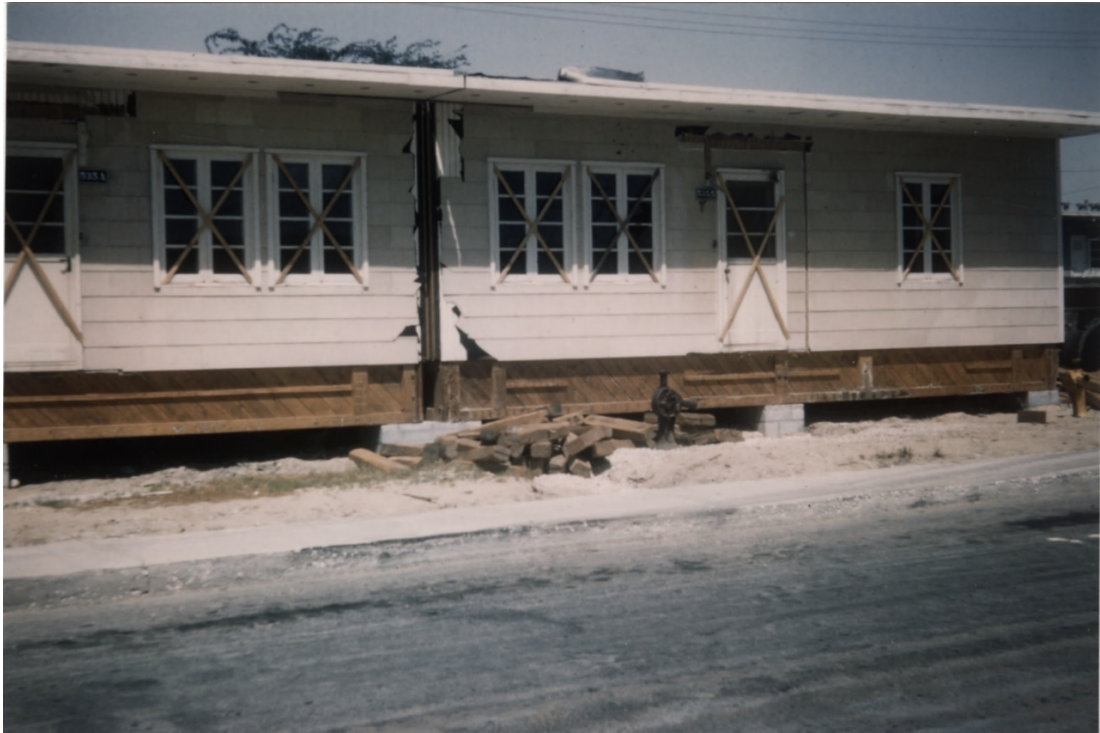
Figure 2.3 A Swedish duplex being prepared for relocating. Photographer unknown. Courtesy of King Abdulaziz Foundation for Research and Archives (Darrah).
