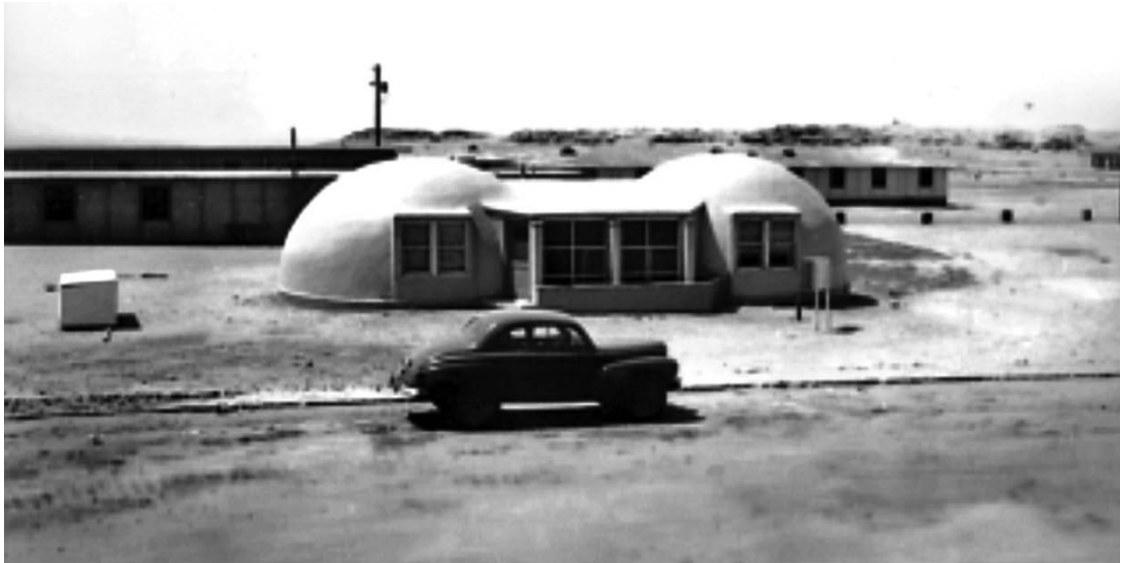
Figure 1.7 Bubble House built in the Dhahran Camp in 1945. The house had two bedrooms and a circular plan living room. Acoustic and insulation issues were the main reasons for the project failure. Photograph by George Fobes. Courtesy of Saudi Aramco.
