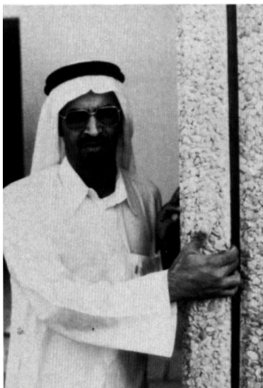
Figure 5.20 Ministry supervisor inserting his fingers in the invisible panel joint. Photo: Allan Kenney.
