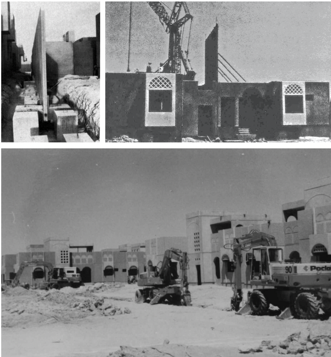
Figure 5.21 Prototype villas under construction. Source: Allan Kenney and REDF Buraidah.
