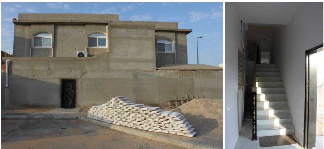
Figure 6.17 Staircase blocking light and air on the house's ground floor. Photos by author.
