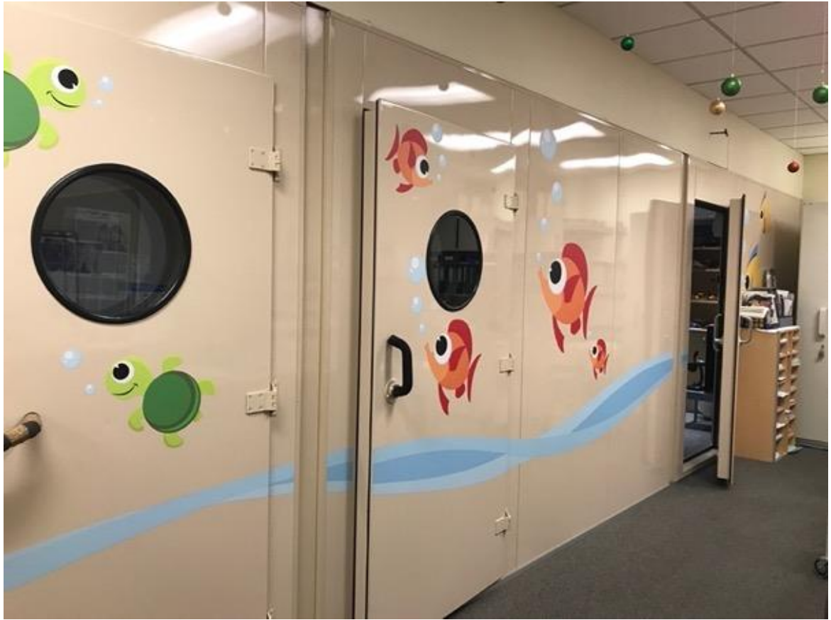
Figure 7: Soundproof booths in an audiology and cochlear implant clinic. Thick, heavy doors decorated with underwater imagery create a subterranean feeling.
