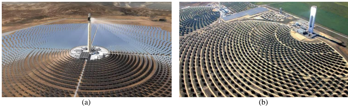
Figure 2.9. Different layouts of a heliostat field. (a) A radial heliostat field, Noor III in Morocco. Image from www.masen.ma , (b) a polar heliostat field, PS10 in Spain. Image from www.eusolaris.eu .
