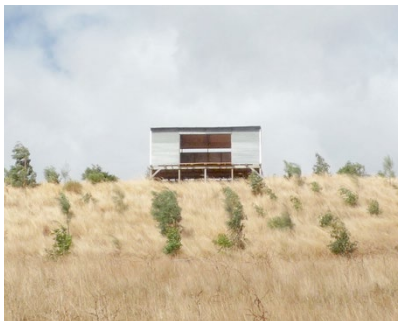
3 The Rural Pavilion , Hay Flat, 2008. Are leisure focused structures awkwardly positioned in Australian culture?
