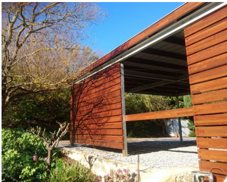
32 This project for a carport in Hay Flat, SA, embodies my ethos for revealed construction and tectonics.
