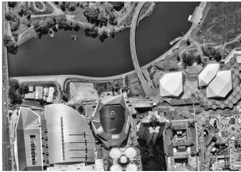
53 Adelaide's congested Riverbank Precinct. Image: Google
