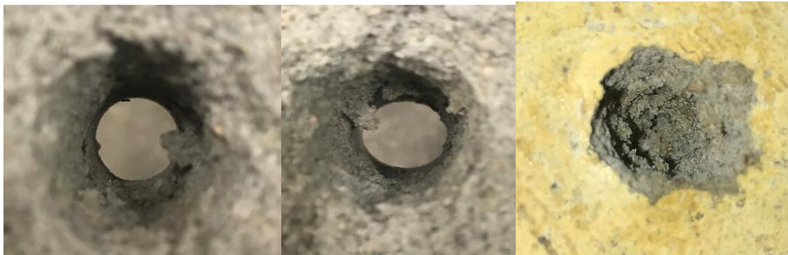
Fig 3. Borehole convergence observed by the camera
