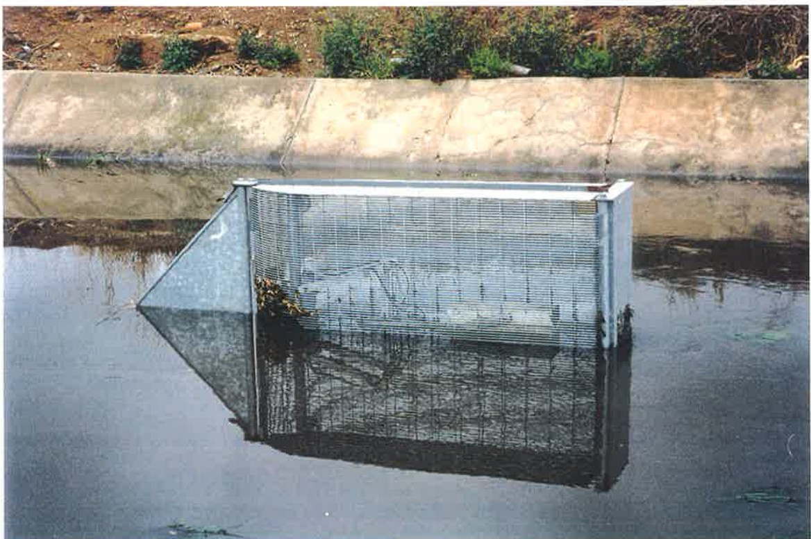
Photograph 5.4 : Storm event after installation of trash racks. Backwatered
