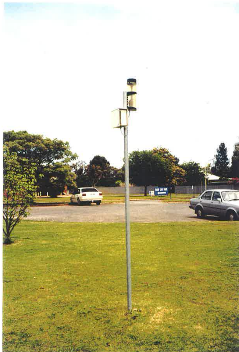
Photograph 4.1 : Hampstead Centre (AU504114) Pluviometer in the Barker Inlet Wetland Catchment
