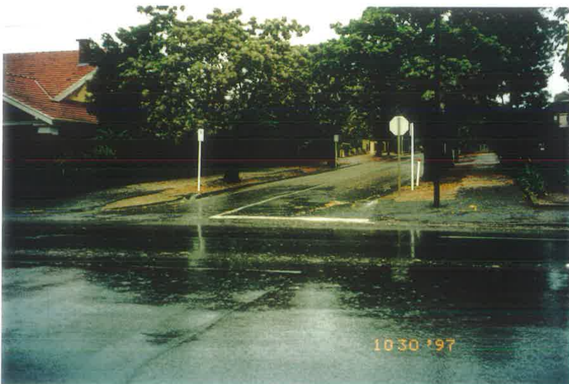
Photograph 3.10 : Typical residential street in The Hindmarsh Enfield Prospect Catchment
