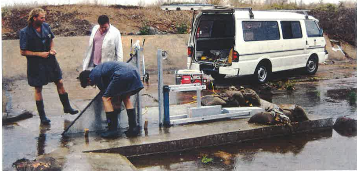
Photograph 4.3 : Construction of the instrument cage.
