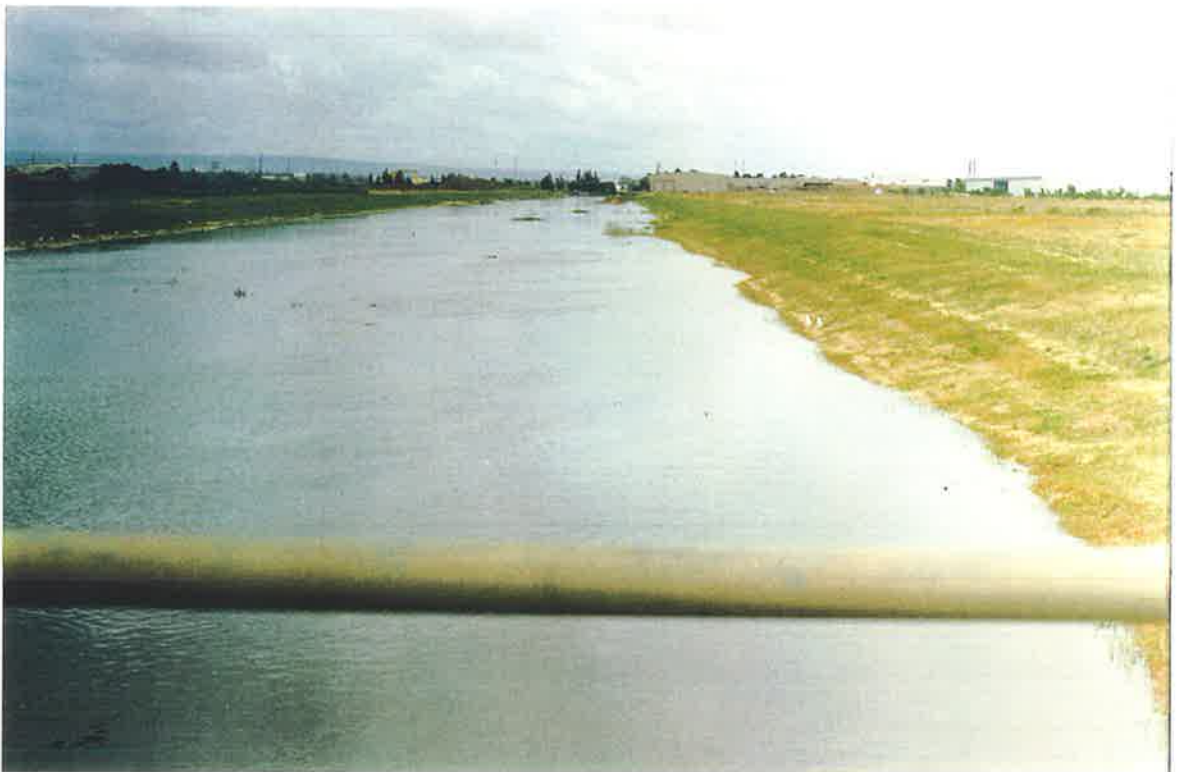
Photograph 3.8 : The swale drain during a storm event. Facing Upstream.
