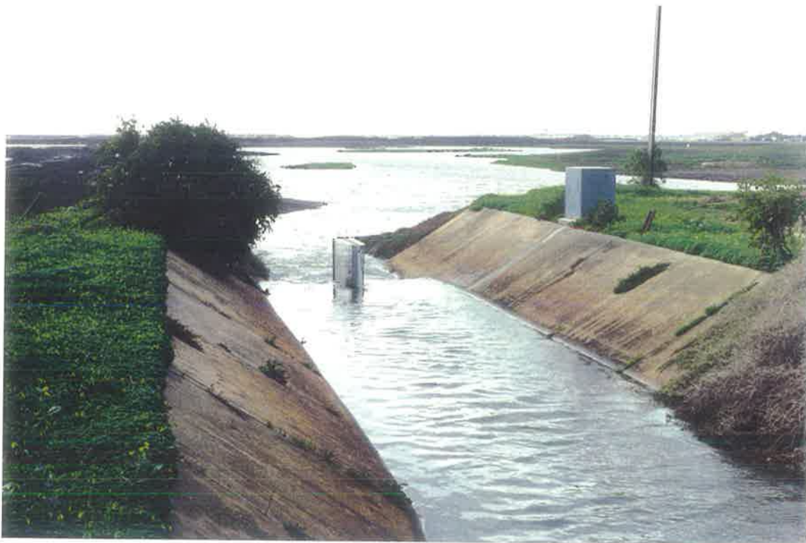
Photograph 3.6 : Facing Downstream of the HEP monitoring station
