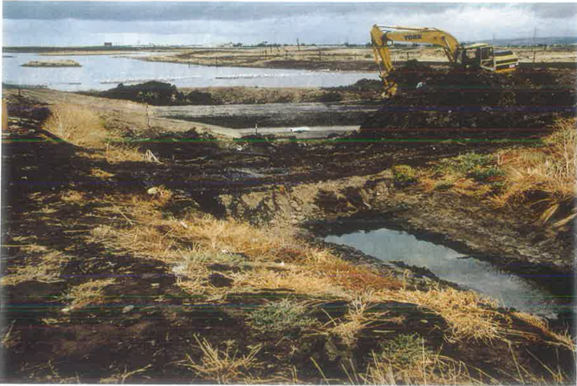
Photograph 4.8 : Construction of trash racks at the HEP Drain.
