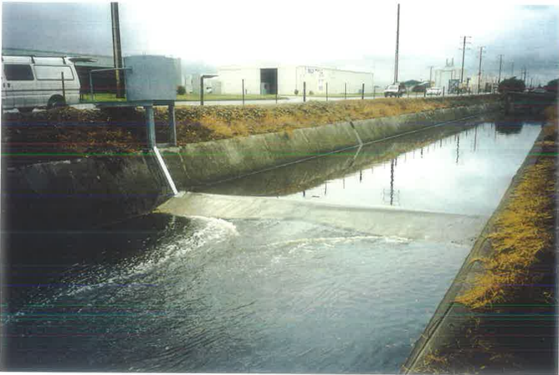
Photograph 3.23 : The monitoring station at the Eastern Parade Drain (AU504201). Facing Upstream.
