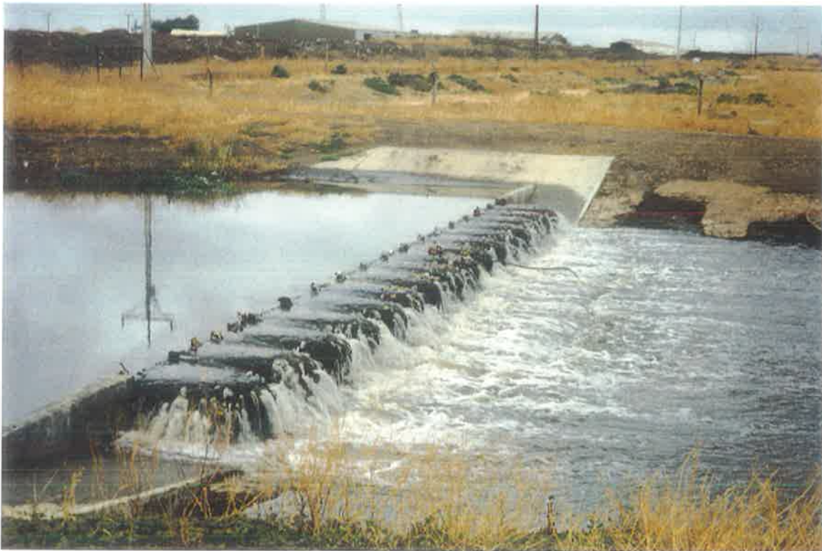
Photograph 4.9 : Trash racks at the North Arm East Drain
