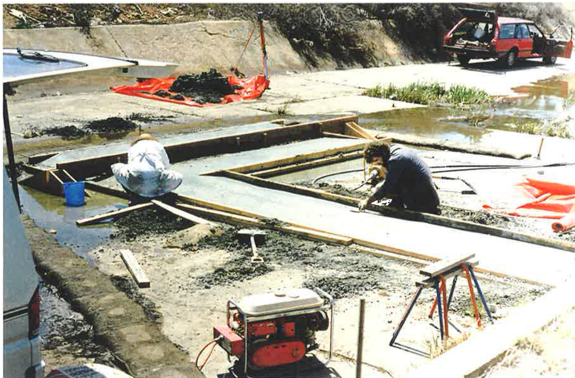
Photograph 4.2 : Construction of the North Arm East Drain Weir
