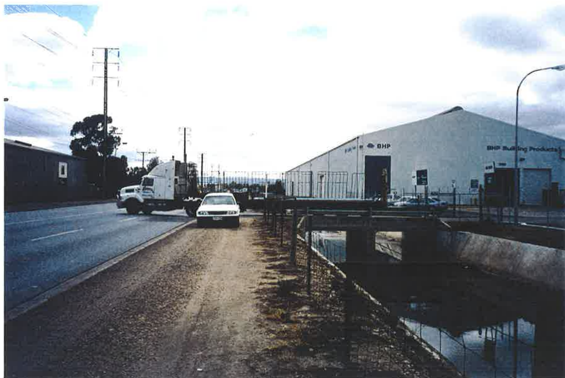
Photograph 3.26 : Typical industrial land use in the The Eastern Parade Catchment (Eastern Parade facing East)
