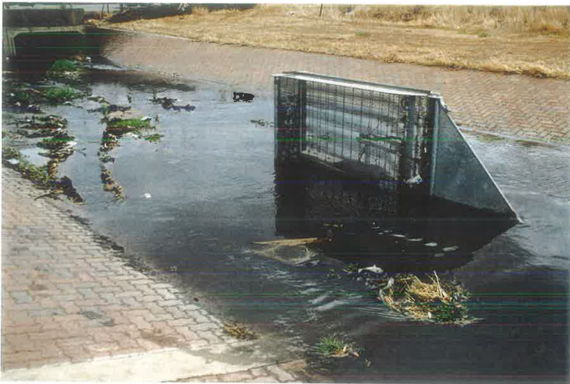
Photograph 3.11 : Dunstan Road Drain (AU504103) monitoring station. Facing downstream.
