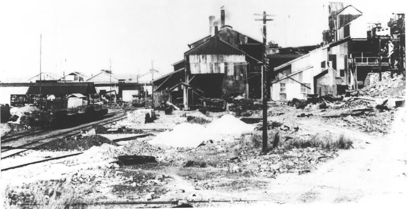
State Smelters Chillagoe, n.d. [1921?] [Photograph courtesy John Oxley Library]
