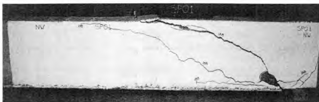
Fig.6.8. Failure of SP01
