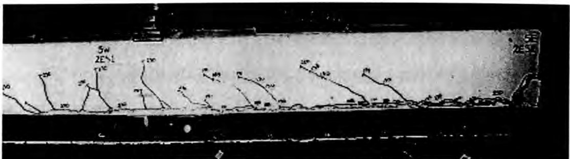
Fig.17.18 (d).Complete debonding of south side plate Fig.17.18. Test-2ES1: Crack patterns
