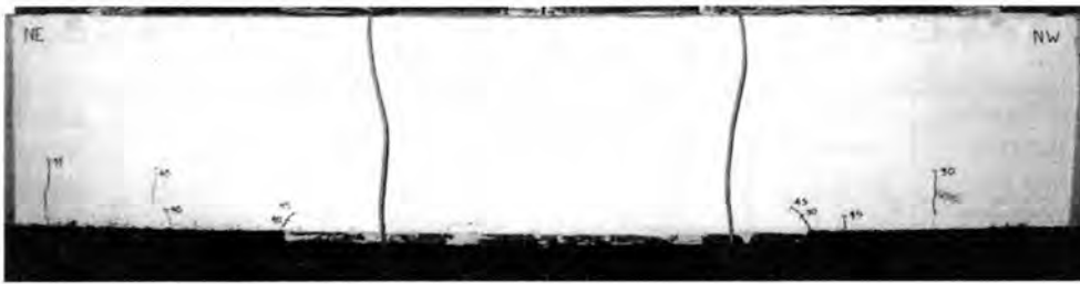
Fig.12.4. FP-T20: Initial flexural crack pattern
