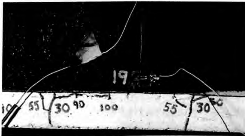
(b) Close view of local debonding crack formation below side plate
