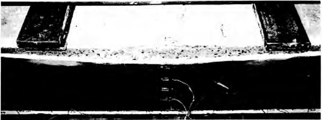
(b) Local buckling and debonding of south side plate
