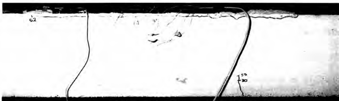
Fig.12.12. Long debonding crack in FP-C20
