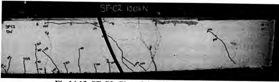
Fig.14.13. SF-C2: Plate debonding on south side
