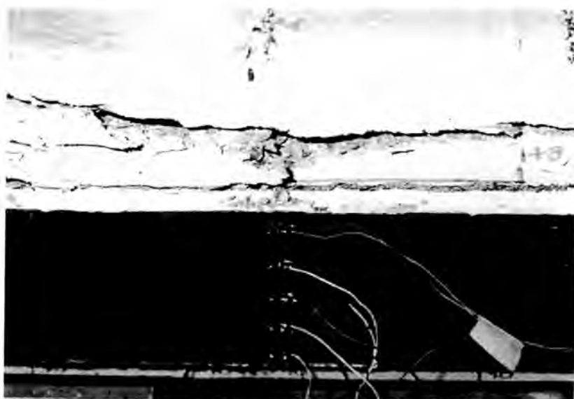
(b) Close view of crushing of concrete and debonding of plate
