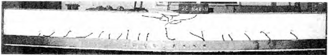
Fig.17.14(b). Overall crack pattern at closure of test
