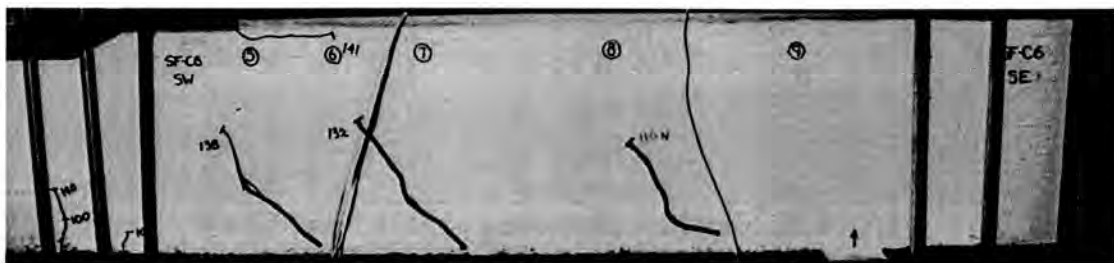
Fig.14.33. Test SF-C6(a): Crack pattern on south side
