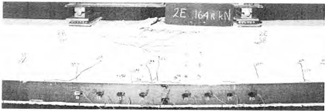
Fig.17.14(d). Concrete crushing in south side
