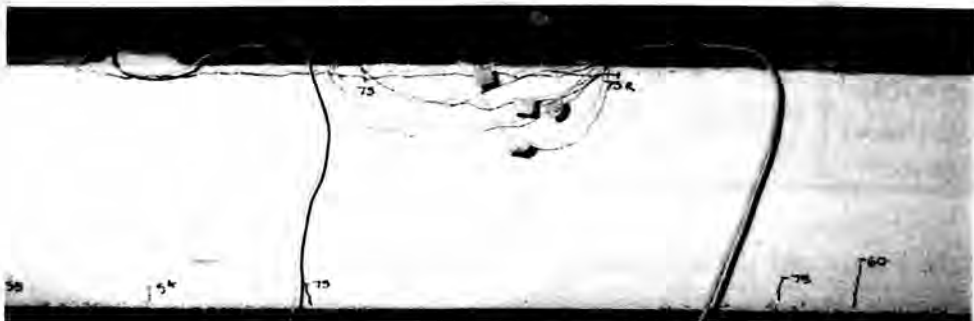
Fig.12.16. Long debonding crack in FP-C25
