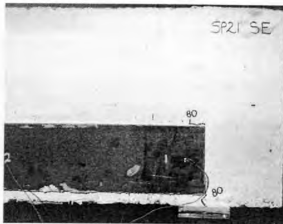
(a) Crack at plate end at P= 80 kN
