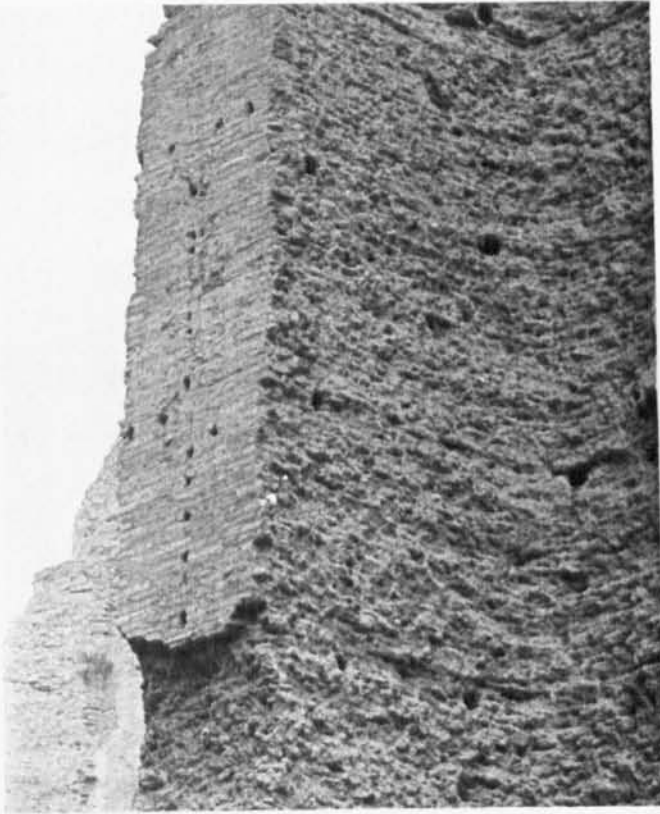
Fig. 127: Baths of Caracalla, central block, Rm 17E, ? holes for fixing window frames.
