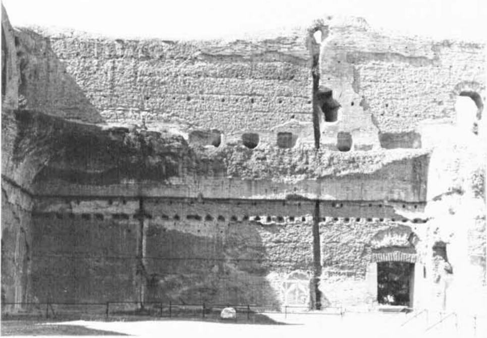
Fig. 64: Baths of Caracalla, central block, Rm 12W, S wall, bonding courses and putlog holes.
