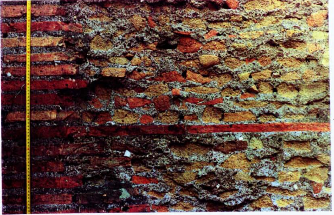
(a) Baths of Caracalla, central block, Rm 3E, brick facing, exposed core and bonding course.
