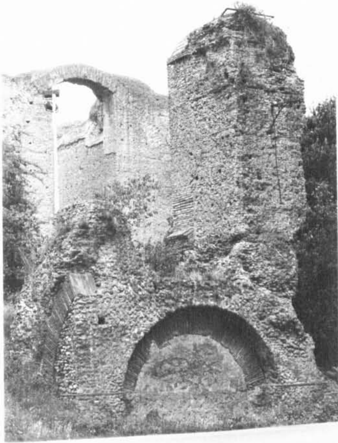
Fig. 3: Baths of Caracalla, remaining pier of N facade.
