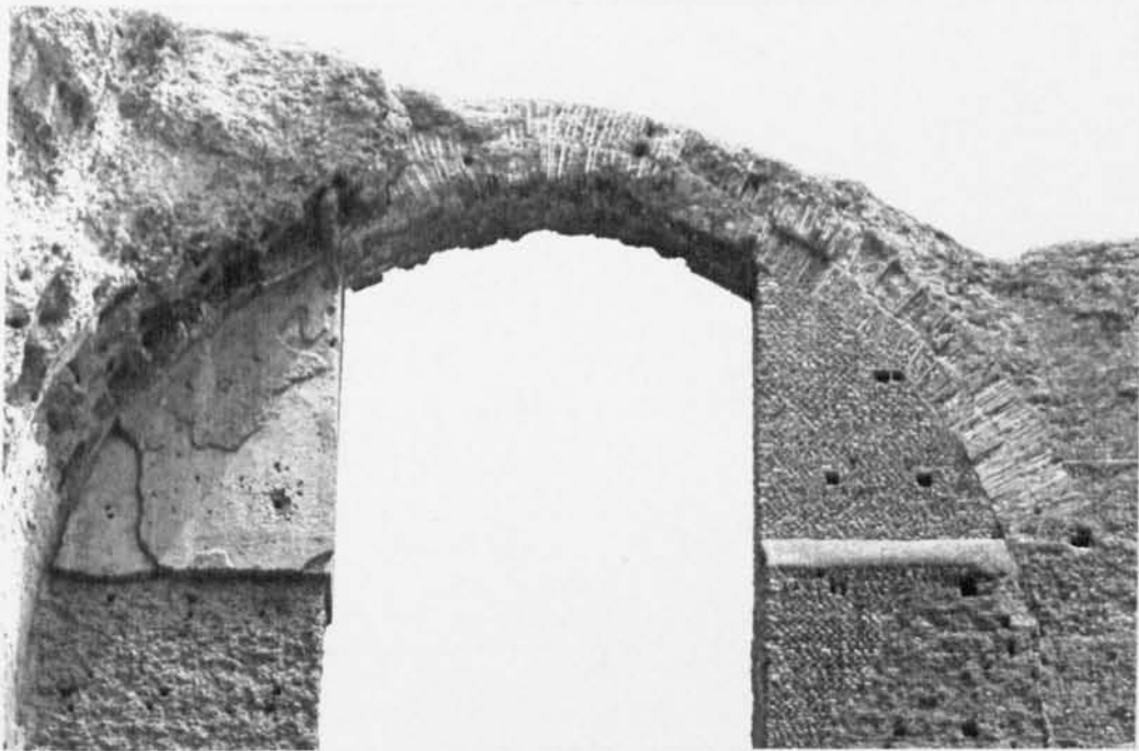
Fig. 94: Baths of Caracalla, central block, Rm 1W, N wall, vault construction.
