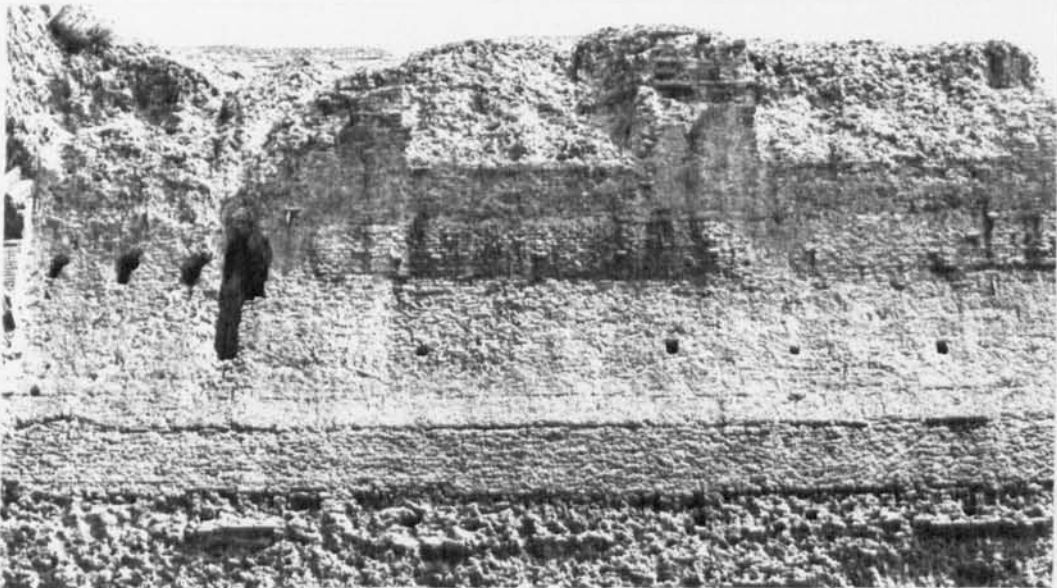
(b) Baths of Caracalla, central block, detail of vault construction as above.
