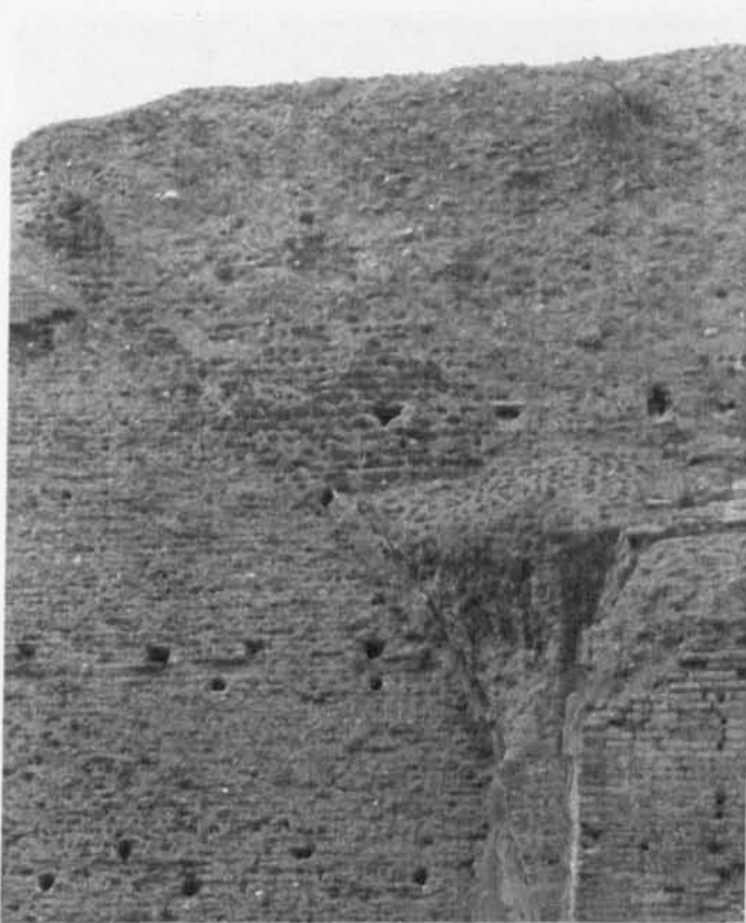
Fig. 88: Baths of Caracalla, central block, Rm 3E, vault construction with pumice in upper levels.
