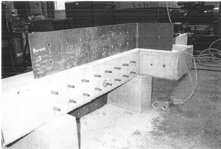
Fig. 9.14 Completion of bolts installation
