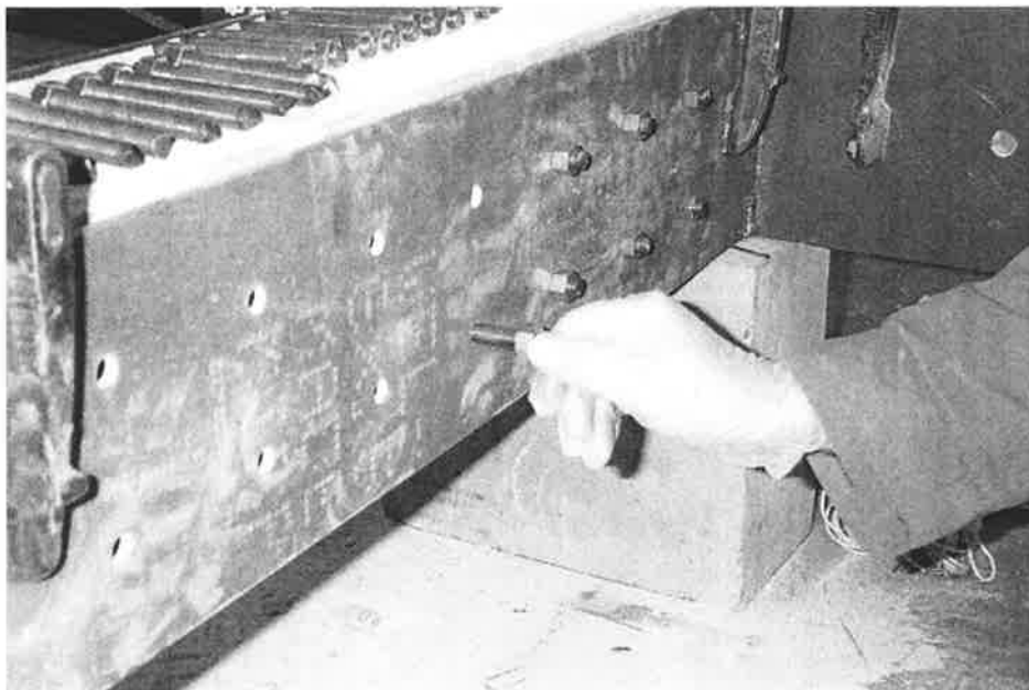
Fig. 9.13 Installation of bolts
