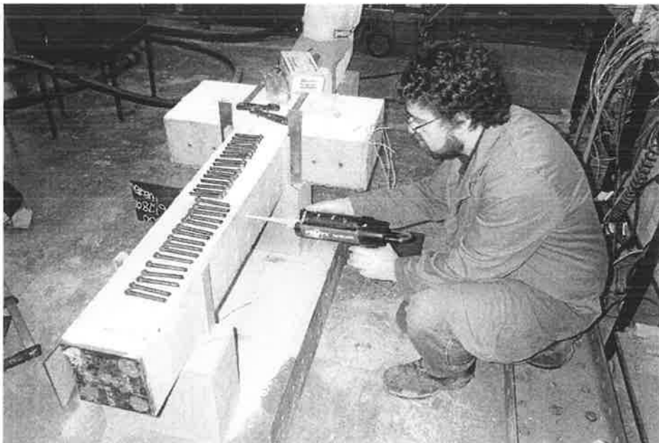
Fig. 9.11 Injection of adhesive
