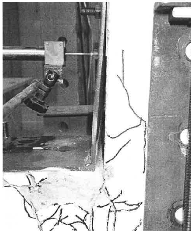
Fig. 11.48 Error in measure point C due to plate lifting up
