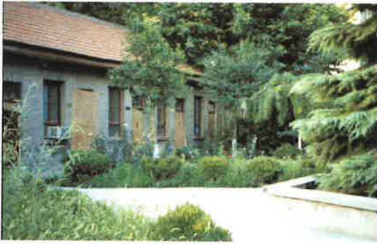
Plate 61: Long Building on Eastern Side of Courtyard, Waiyuan Yiyuan , 2001
