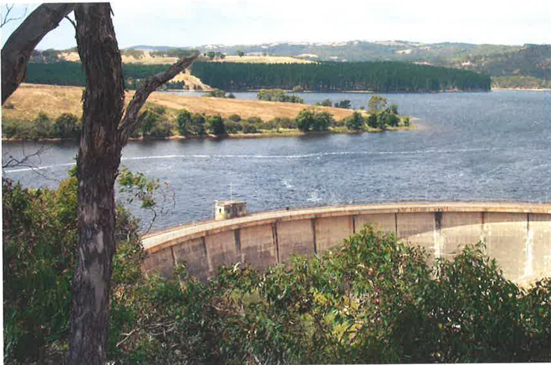
Figure 3.2 Myponga Reservoir, the bubble plume generated by the aerator is visible in the foreground. The off-take tower can be seen atop the dam wall.
