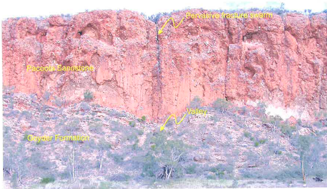
Figure 9.21. The regularly spaced valleys are controlled by pervasive fractures as demonstrated by this example in the Pacoota Sandstone and Goyder Formation at Glen Helen Gorge viewed towards the south. The valleys like the one shown here are mappable from aerial photography.
