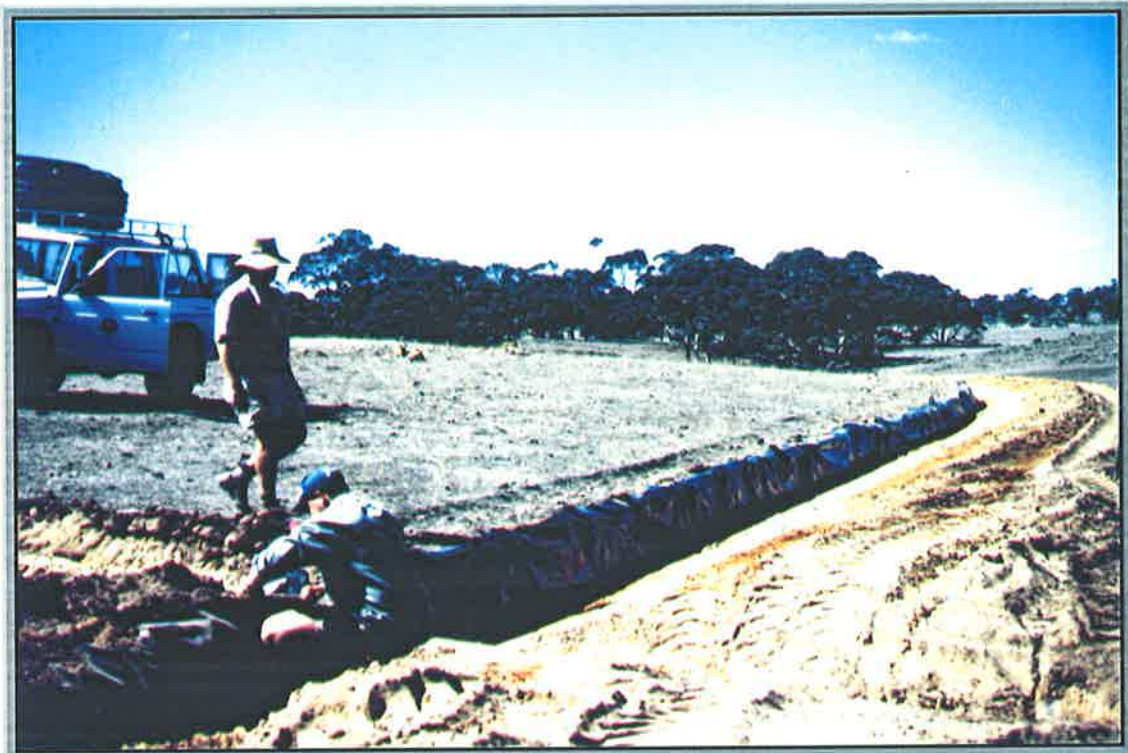
Plate 3.2 Plastic barrier preventing throughflow to lower site.
