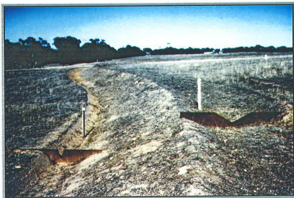
Plate 3.5 V-notch weirs installed on reverse interceptor drain
