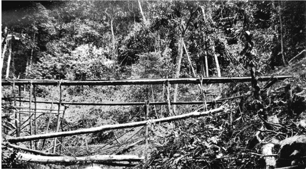
Fluming water across a ravine
