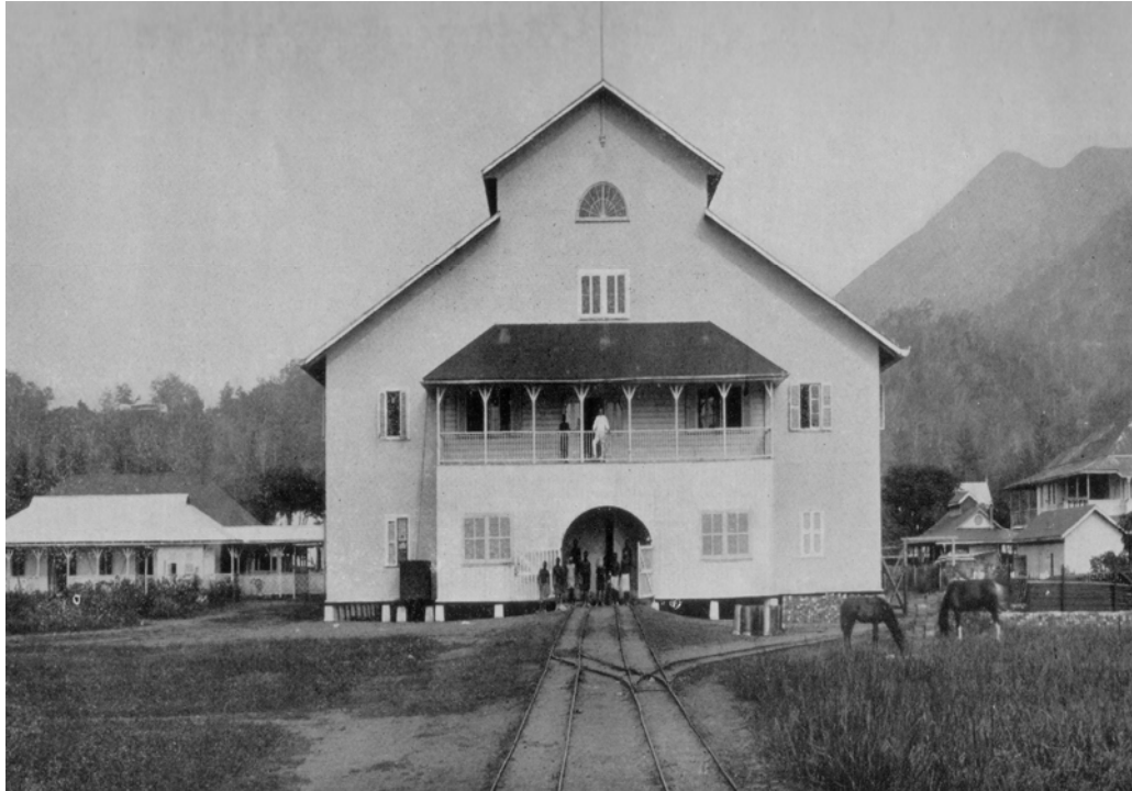
NGC central warehouse Rabaul, c. 1914
