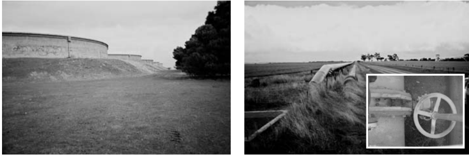
Figures 7-2 and 7-3 – Hanson summit storage tanks and “Sheep Dip” in-line butterfly valve boundaries
