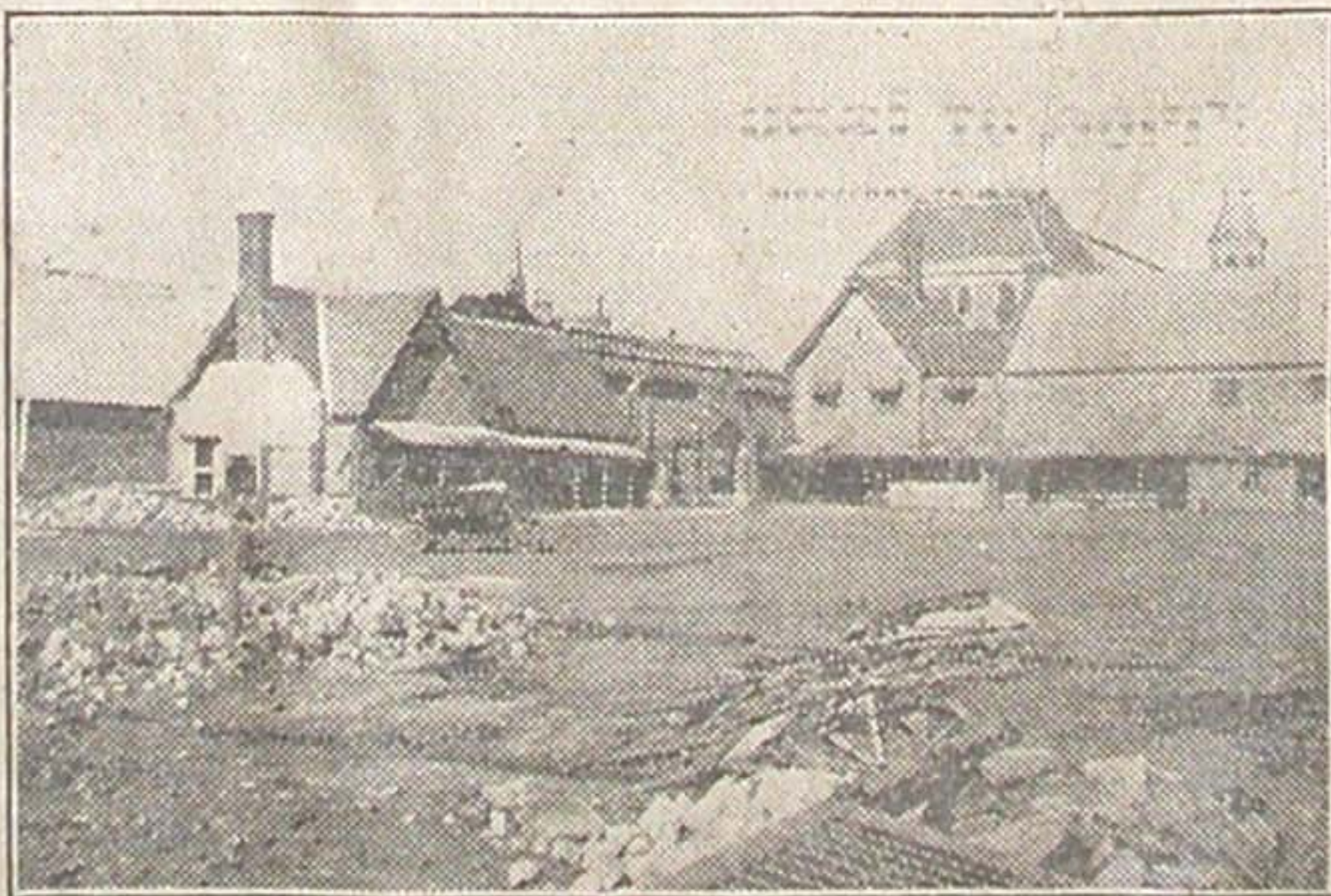
Fast disappearing—the old mounted police barracks on North Terrace in process of demolition to allow of University and Public Library extension.
