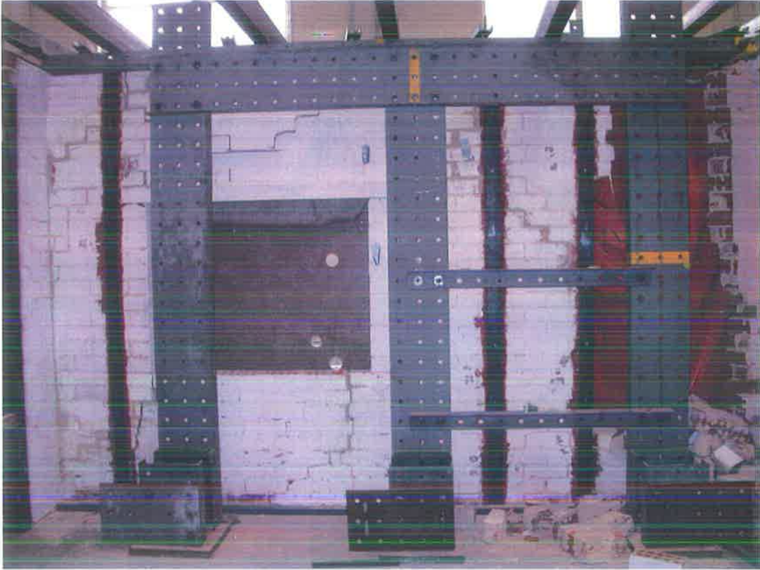
Overall cracking and failure pattern of Wall 3
