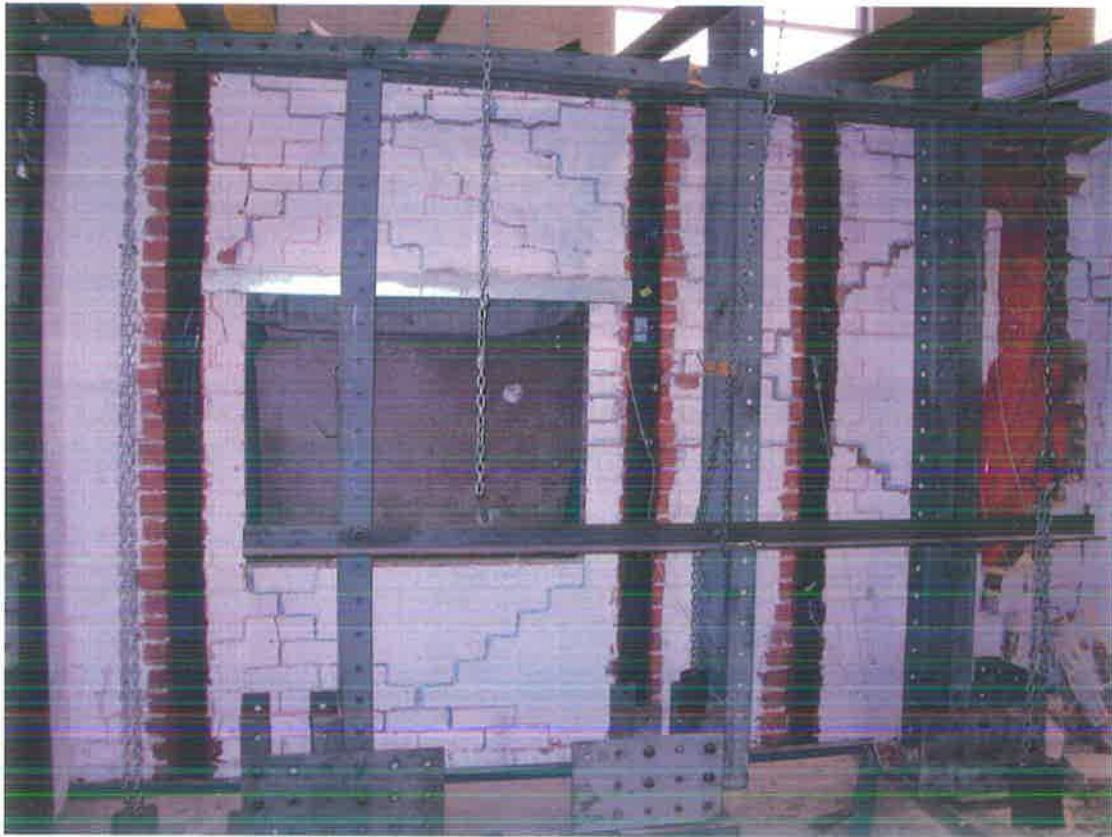
Overall cracking and failure patterns of Wall 2
