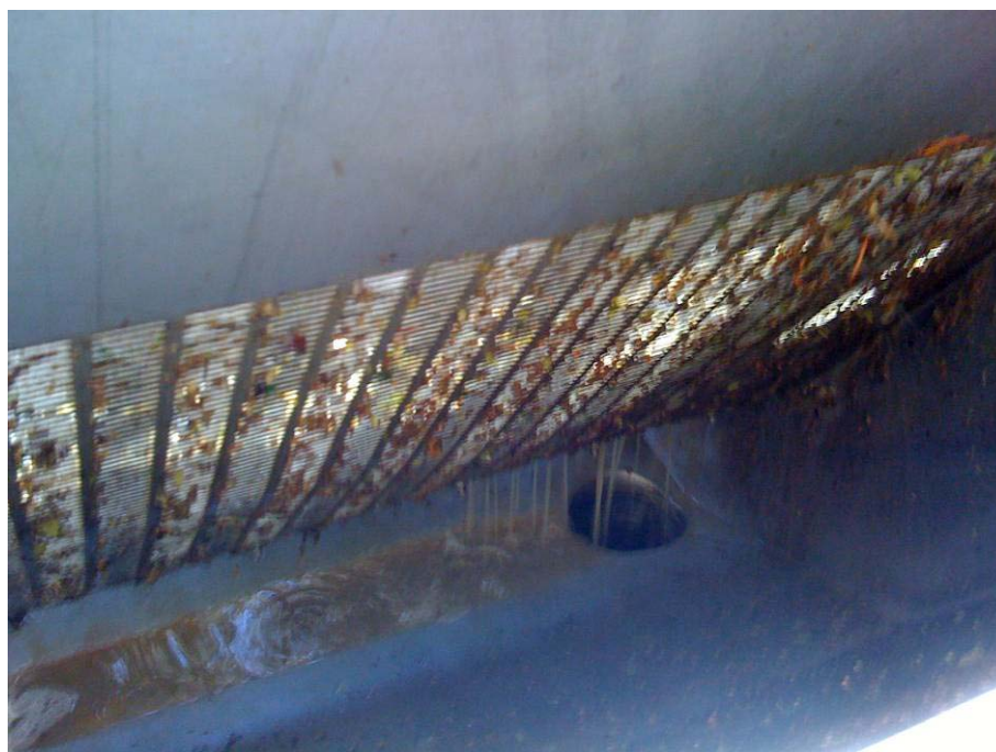
Figure 7.5: Underside of draining section at feed to destemmer-crusher (drain hole to buffer tank shown)
