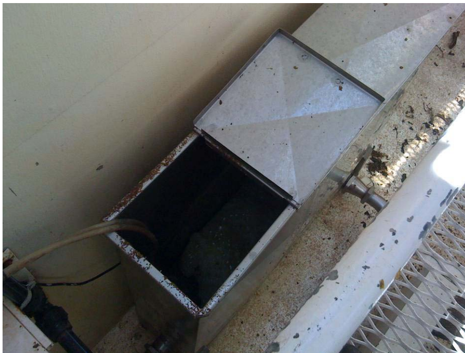
Figure 7.6: Buffer tank for destemmer-crusher run-off
