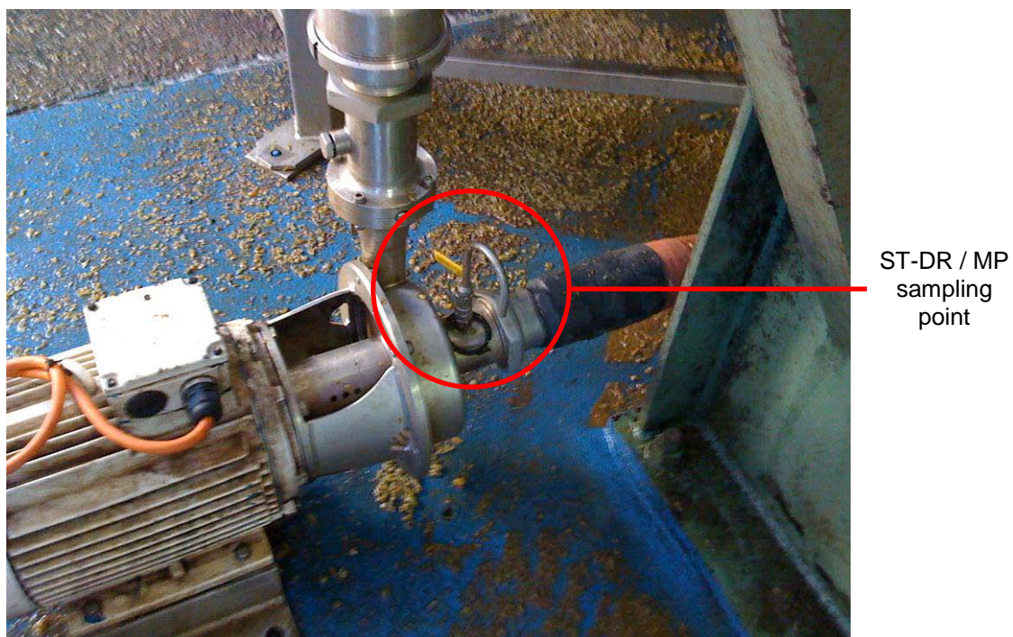
Figure 7.16: Sample tap immediately downstream of static drainer and membrane press buffer tanks
