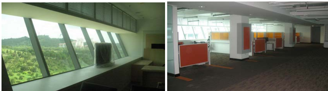
Left: Facade lightshelf with fixed louvers for glare prevention; Right: Facade daylight seen from a corridor
