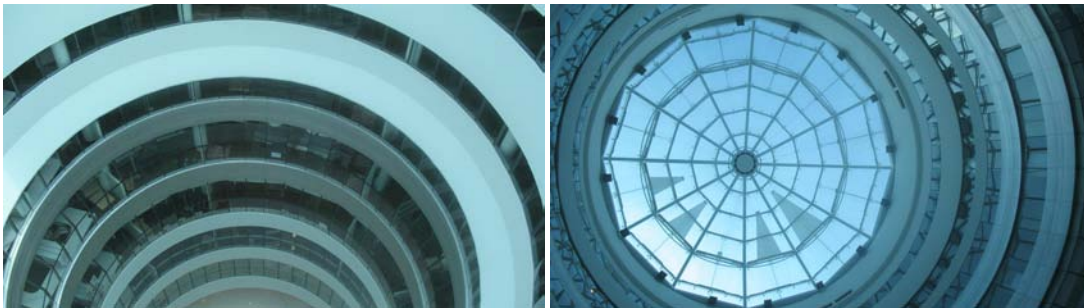
Left: Atrium looking downward; Right: Atrium looking upward
