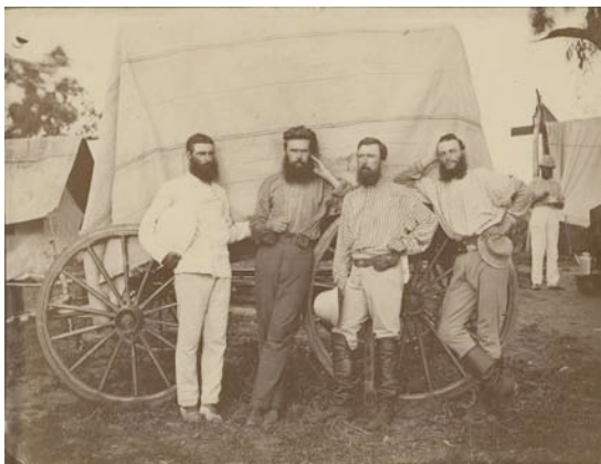
Plate 127 Overland Telegraph construction party 11 March 1872, Roper Depot, NT
