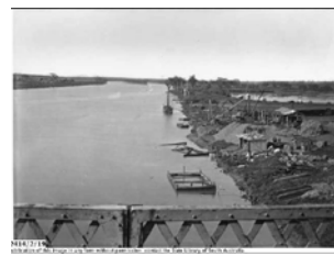
Bridge Building, Murray Bridge 1873-79, Murray Bridge SLSA B 62414/2/19 SWS.6.093.02 [2] 410
