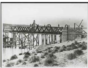
Bridge Building, Murray Bridge 1873-79, Murray Bridge SLSA B 18558 SWS.6.094.01 [1] 408
