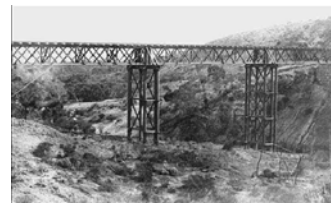
Lattice Bridge June 1882, Pichi Richi Pass (near Quorn) SLSA B 62381 SWS.3.006.02 [2] 324
