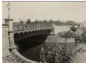
City Bridge 1877-85, Adelaide SLSA B 7303 SWS.8.176.01 [1] 418
