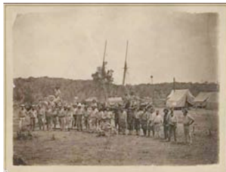
Darwent and Dalwood's OT Line Construction Team at Southport Sept 1870, Southport SLSA B 9763 SWS.1.042.01 [2] 89
