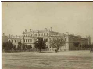
Government Offices [Torrens Building] 1883-85, Adelaide SLSA B 7492 SWS.8.151.02 [3] 933
