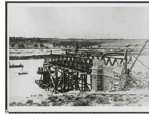
Bridge Building, Murray Bridge 1873-79, Murray Bridge SLSA B 18565 SWS.6.095.01 [1] 407
