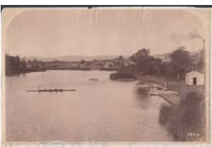
Boat house, River Torrens 1881-85, Adelaide Private Collection SWS.8.211.01 [1] 544
