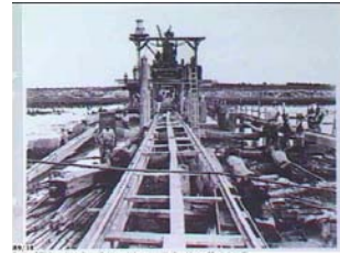
Murray Bridge Construction 1873-79, Murray Bridge SLSA B 17389/38 SWS.6.084.01 [1] 413
