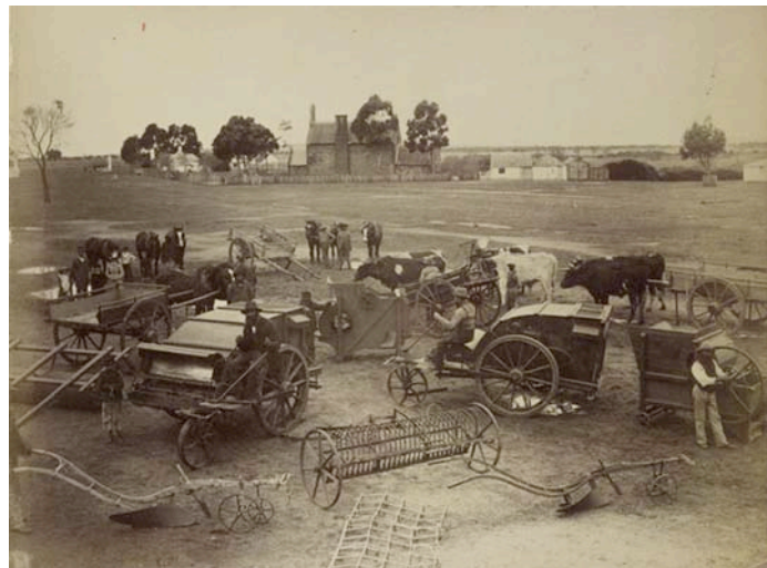
Plate 129 Poonindie Mission, South Australia 1884, Poonindie
