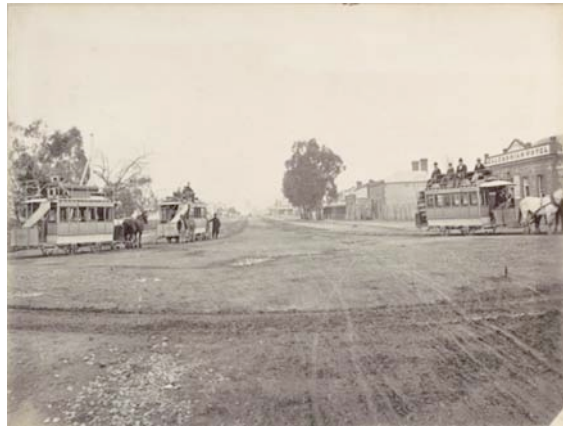
Plate 145 Adelaide & Suburban Tramway Co. Terminus at O'Connell Street [aka O'Connell Street] c.1879 (1878-80), North Adelaide
