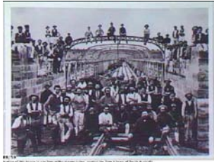
Bridge Workers, Murray Bridge 1877-79, Murray Bridge SLSA B 17389/59 SWS.6.089.01 [1] 414
