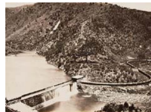
Weir and Pipe 1866-85, Torrens Valley NLA nla.pic-an20886593-69 SWS.6.113.01 [5] 445
