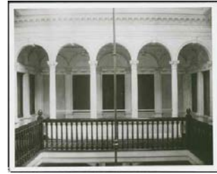
Picture Gallery columns, Martindale Hall 1880-85, Mintaro SLSA B 17732/5 SWS.10.052.01 [1] 768
