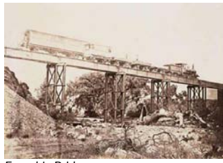
French's Bridge June 1882, Pichi Richi Pass (near Quorn) NLA nla.pic-an20886593-40 SWS.3.005.01 [4] 326
