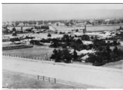
North Adelaide View [from Stanley Street] 1 st section 1872-81, North Adelaide SLSA B 6418 SWS.9.011.01 [2] 917
