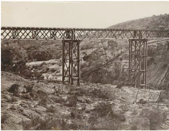
Plate 137 Lattice Bridge at Saltia Creek 1882, Pichi Richi Pass (near Quorn)
