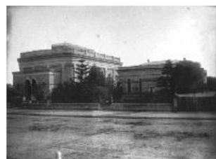
Tynite Street Baptist Chapel 1875-85, North Adelaide AGSA 991Ph1.16 SWS.8.147.01 [1] 509
