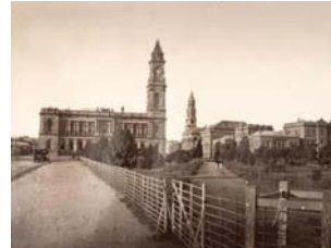
View from Victoria Square, Adelaide 1876-82, Adelaide AGSA 991Ph1.33 SWS.8.161.02 [4] 853
