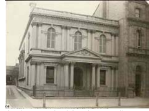
Savings Bank of South Australia 1866-85, Adelaide SLSA B 2920 SWS.8.073.01 [1] 962
