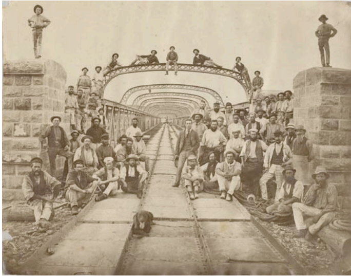
Plate 136 Bridge Workers, Murray Bridge 1877-79, Edwards Crossing [Murray Bridge]
