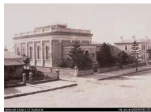
Baptist Church, Tynite Street 1875-85, North Adelaide NLA nla.pic-an20886593-55 SWS.8.145.01 [1] 510
