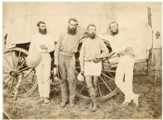
Plate 128 Overland Telegraph construction party 11 March 1872, Roper Depot, NT
