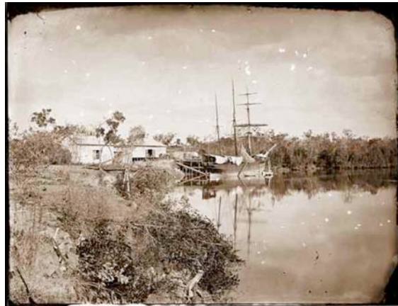
Plate 116 Southport Jetty showing the Estelle September 1870, Darwin
