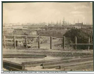
Port Adelaide Dock 1879, Port Adelaide SLSA B 10743 SWS.5.026.01 [1] 248
