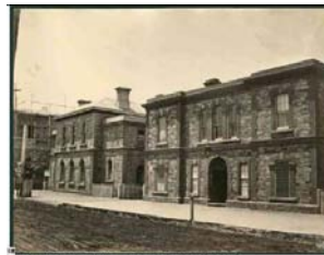
Post Office, Port Adelaide 1879, Port Adelaide SLSA B 10738 SWS.5.029.01 [1] 227
