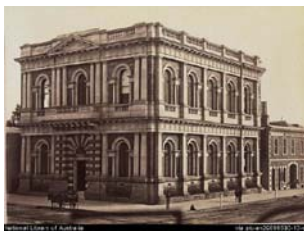
Bank of Adelaide 1880-82, Adelaide NLA nla.pic-an20886593-13 SWS.8.175.02 [3] 957
