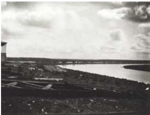
Girders awaiting assembly for Murray Bridge 1868-73, Murray Bridge NGA 86.1855 SWS.6.088.02 [2] 405
