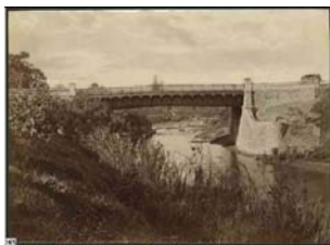
City Bridge 1877-85, Adelaide SLSA B 13265 SWS.8.067.01 [3] 420
