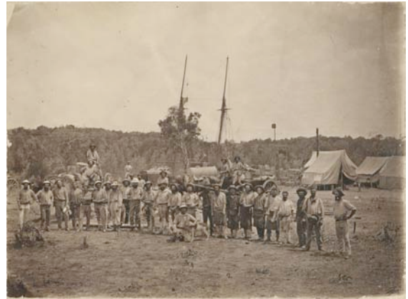
Plate 113 Darwent and Dalwood's OT Line Construction Team at Southport September 1870, Southport
