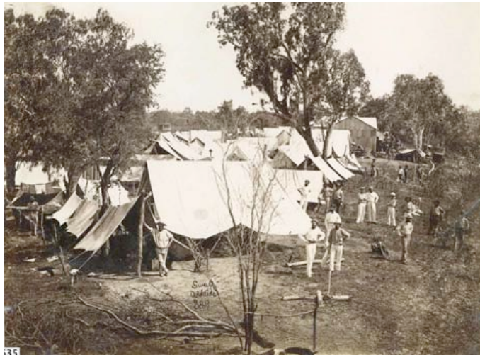
Plate 126 Roper River camp 11 March 1872, Roper Depot, NT
