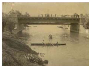
City Bridge 1877-85, Adelaide SLSA B 8868 SWS.8.177.01 [4] 421
