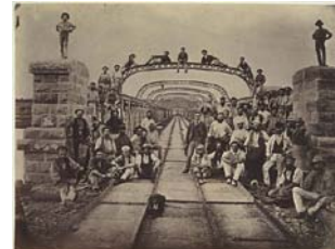
Bridge Workers, Murray Bridge 1878-79, Murray Bridge NGA 89.1594 SWS.6.090.02 [2] 416
