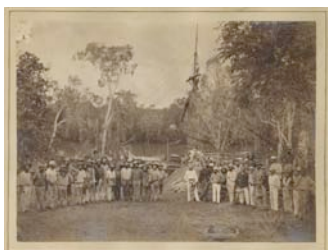
Roper River Jetty 11 March 1872, Roper River, NT SLSA B 9762 SWS.1.038.01 [3] 106
