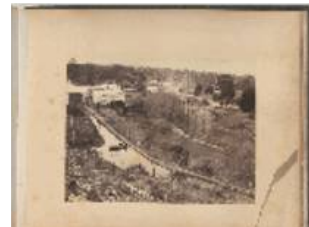
Dunn & Co. Mill Bridgewater [aka Cox's Creek] 1877-78, Bridgewater NGA 2007.81.121.27 SWS.6.211.01 [1] 121
