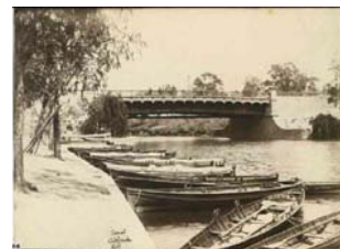
City Bridge 1881-85, Adelaide SLSA B 3566 SWS.8.179.01 [1] 422
