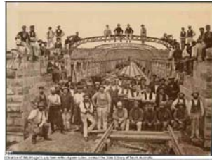
Bridge Workers, Murray Bridge 1877-79, Murray Bridge SLSA B 11708 SWS.6.091.01 [2] 415
