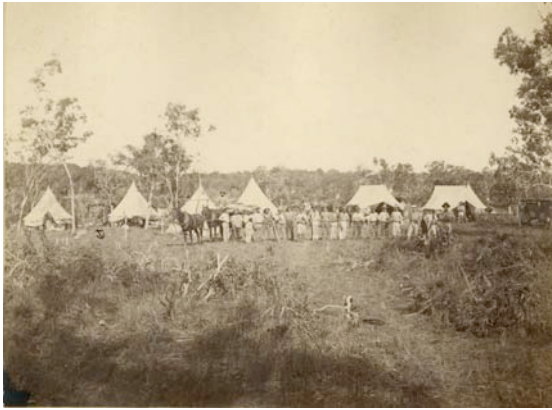
Plate 112 Darwent and Dalwood's OT Line Construction Team at Southport September 1870, Southport
