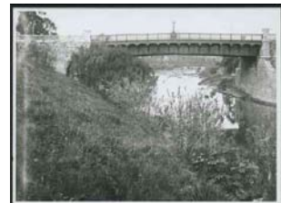
City Bridge 1877-85, Adelaide SLSA B 21716 SWS.8.178.01 [1] 419
