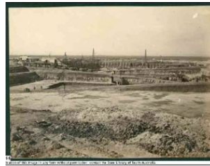
Port Adelaide Dock 1879, Port Adelaide SLSA B 10744 SWS.5.027.01 [1] 247
