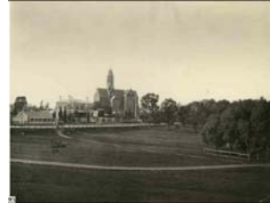
Pennington Terrace, North Adelaide 1876-85, North Adelaide SLSA B 2895 SWS.9.022.01 [1] 516
