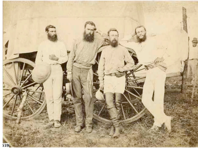
Plate 23 Overland Telegraph construction party 1872, Roper River, NT
