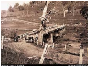
Ledgard's Bridge 1871-85, near Gumeracha NLA nla.pic-an20886593-65 SWS.6.201.01 [1] 435
