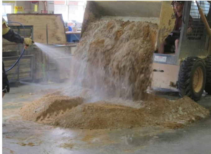
Figure 2 Mixing process of cement-earth mixture
