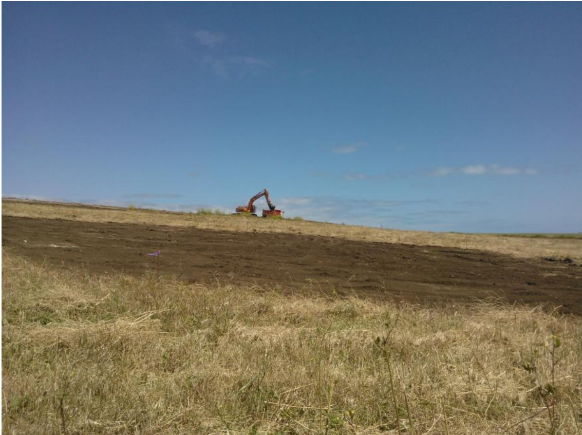
Figure 43. Preparation for development underway at Seaford Heights
