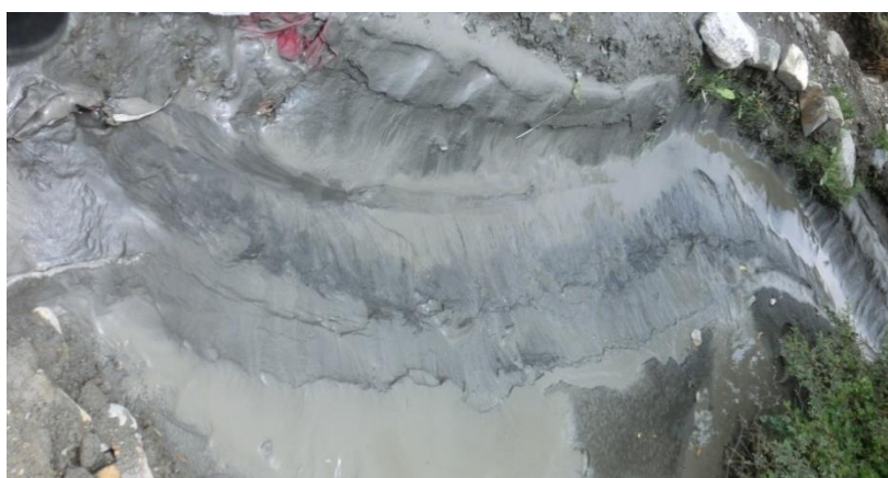
b. Highly silted irrigation infrastructure in the Trans-Himalaya, Nepal
