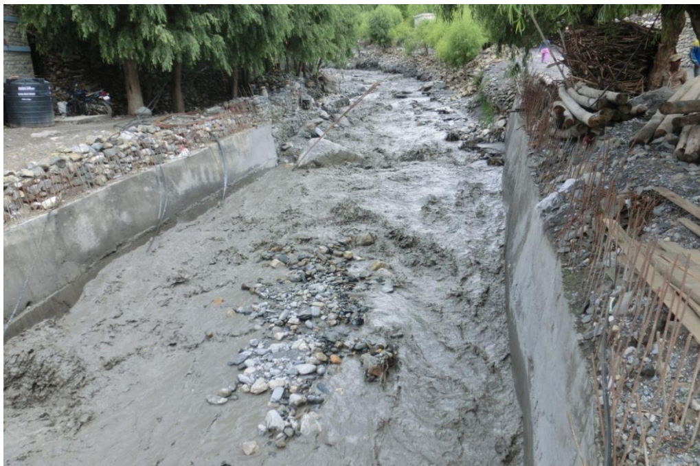
Plate 6.4: Flood Control through Concrete wall in the Trans-Himalaya, Nepal (Source: Field Survey, 2013)
