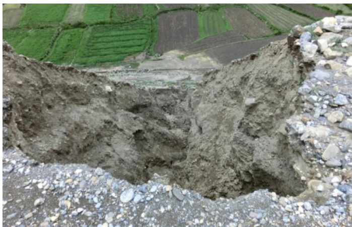
b. Haphazard Construction of Mountain Road is Causing Heavy Landslides in the Trans-Himalaya
