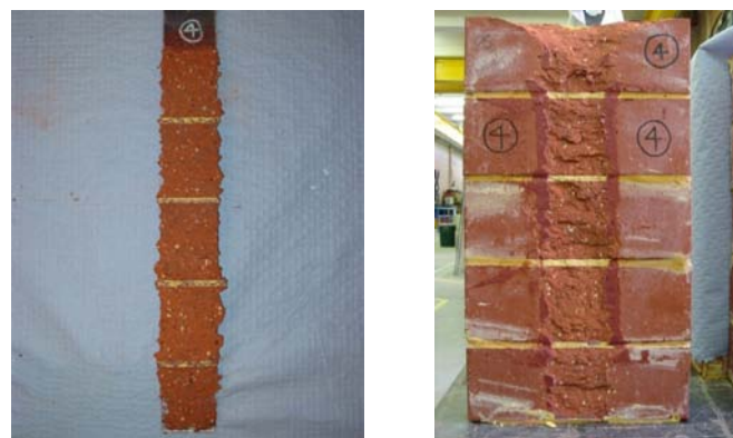
Figure 4.6 GFRP fully debonding failure
